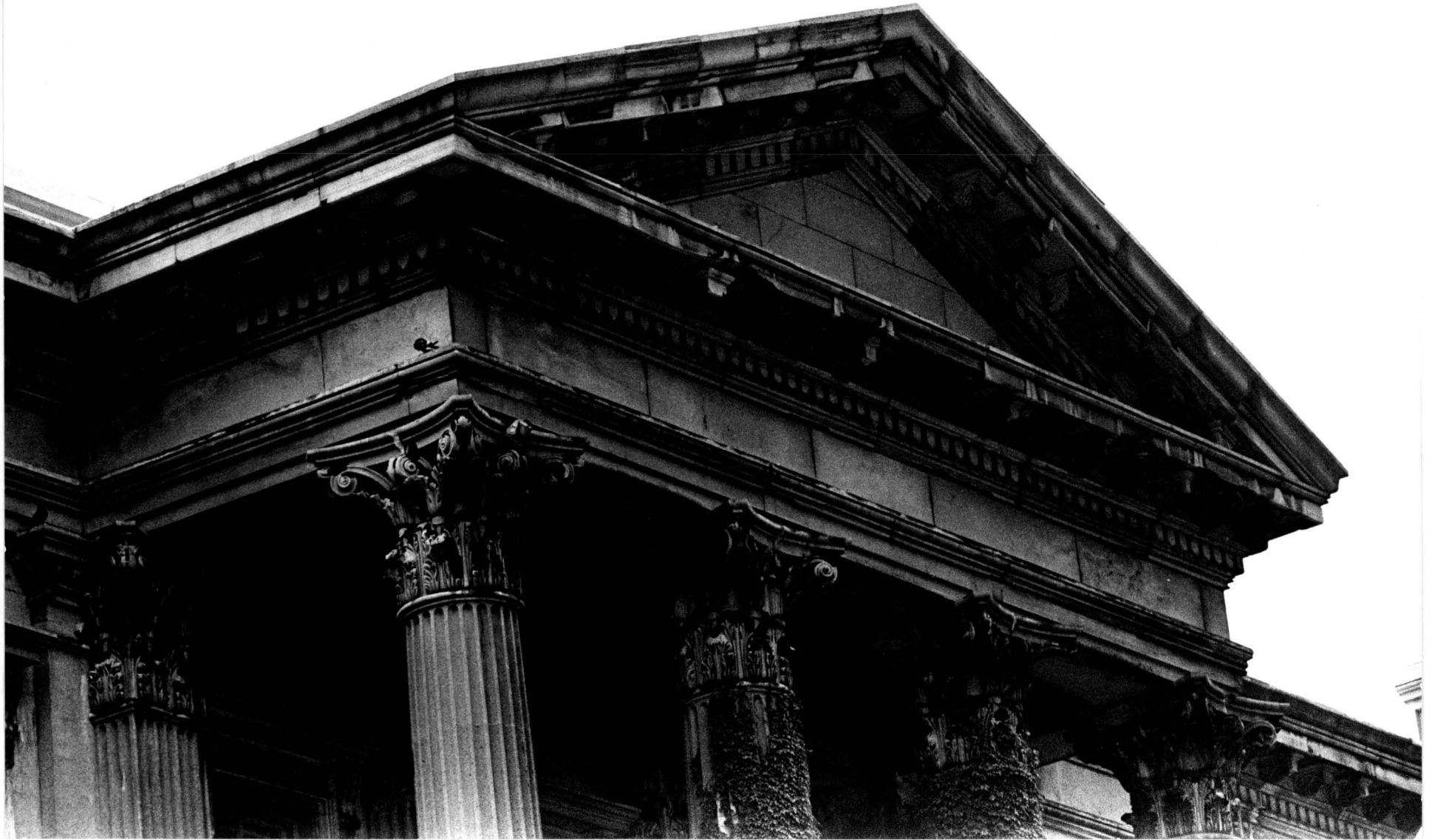
TWEED COURTHOUSE, detail Chambers Street facade
