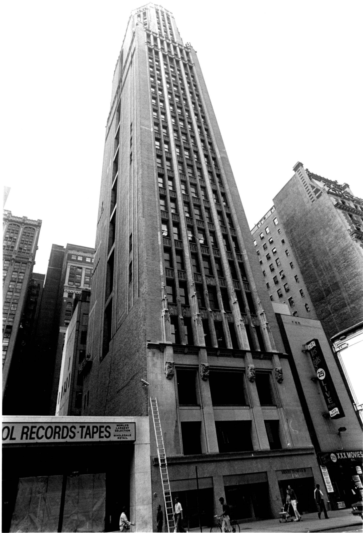
The Bush Tower, 130-132 West 42nd Street and 133-137 West 41st Street 1916-1918, added to in 1921; Helmle & Corbett, Architects 42 Street Facade
