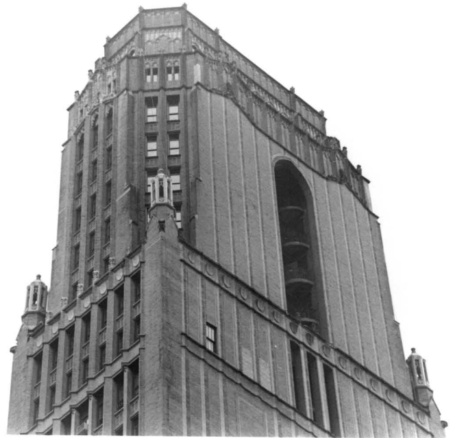
The Bush Tower, 130-132 West 42nd Street and 133-137 West 41st Street 1916-1918, added to in 1921; Helmle & Corbett, Architects
