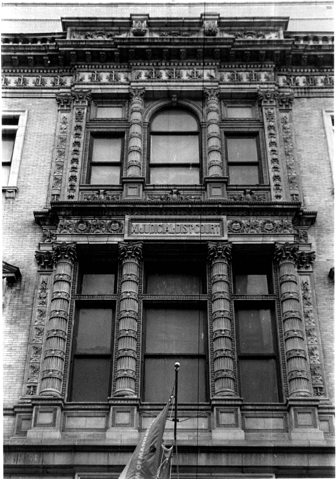
Former Eleventh Judicial District Courthouse 314 West 54th Street; detail, 54th Street facade John H. Duncan, architect; built 1894-96
