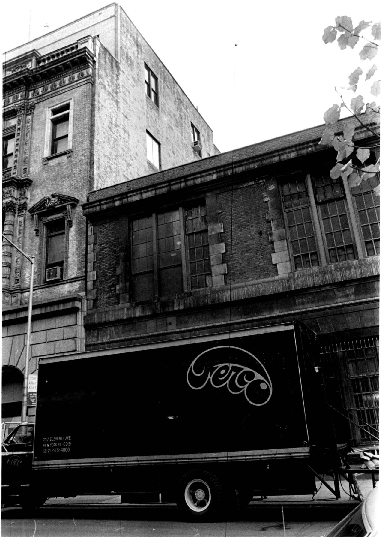
Former Eleventh Judicial District Courthouse 314 West 54th Street; West facade John H. Duncan, architect; built 1894-96
