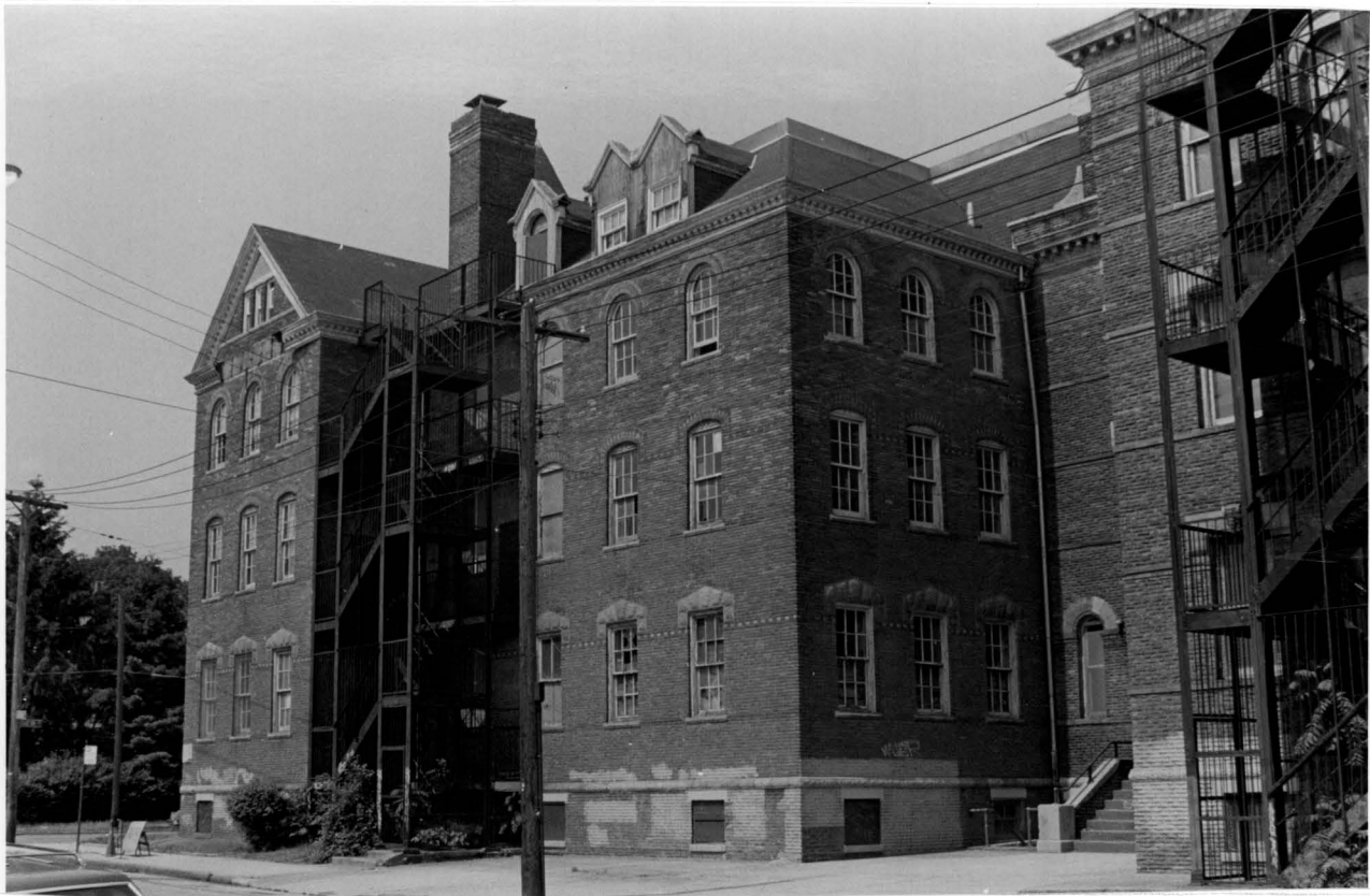
P.S. 20 Annex Heberton Avenue elevation (east) of the 1891 building Photo: Carl Forster
