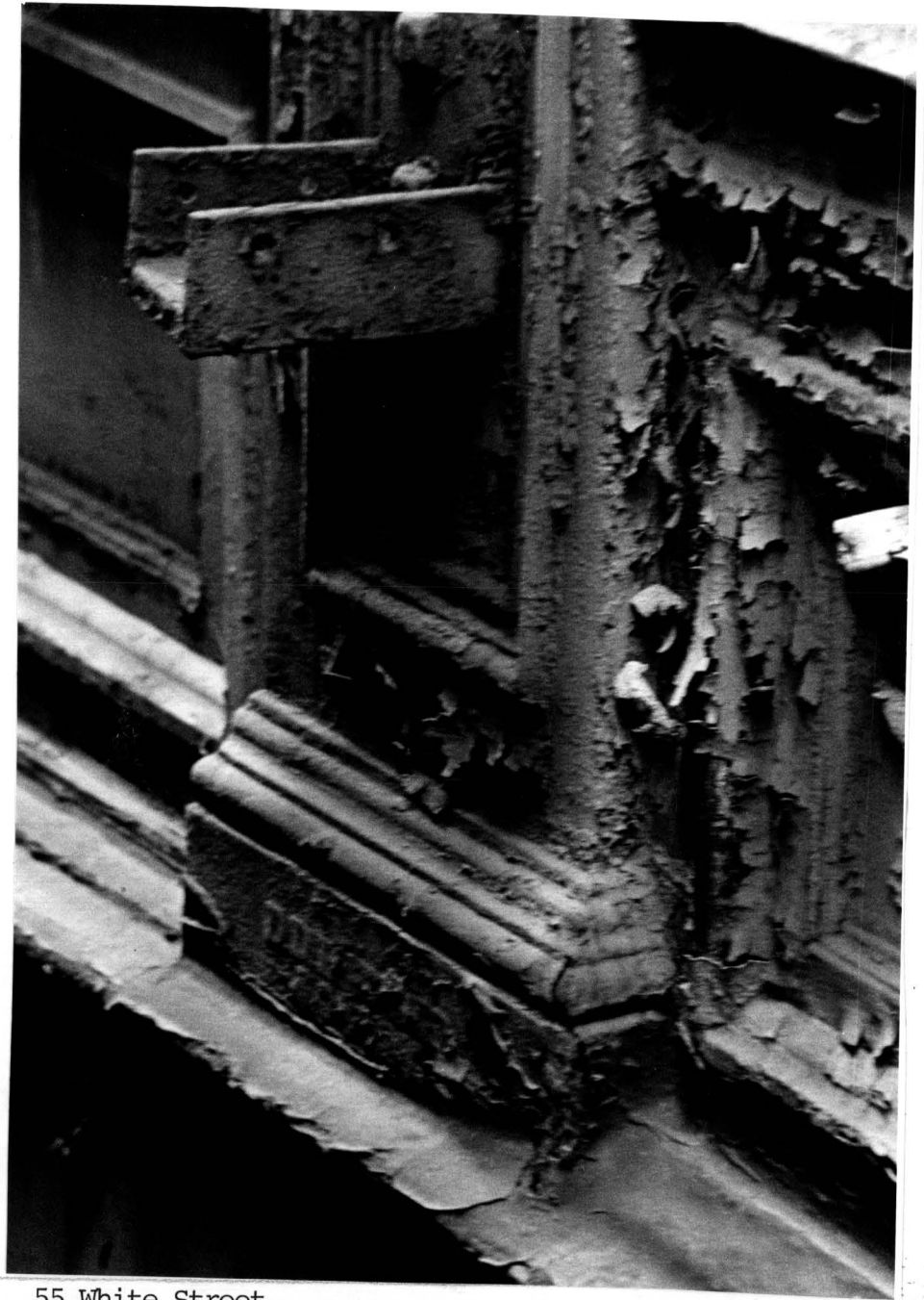
55 White Street Detail of foundry plate with "D. D. Badger" Photo: Carl Forster
