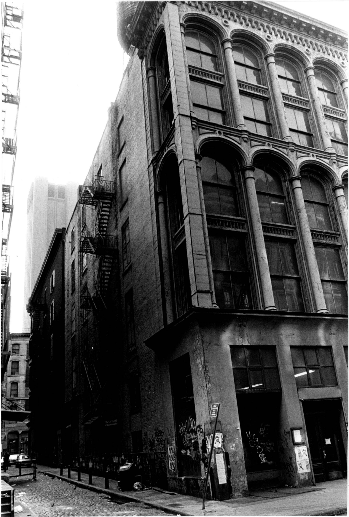
55 White Street View of the White Street and Franklin Place elevations Photo: Carl Forster
