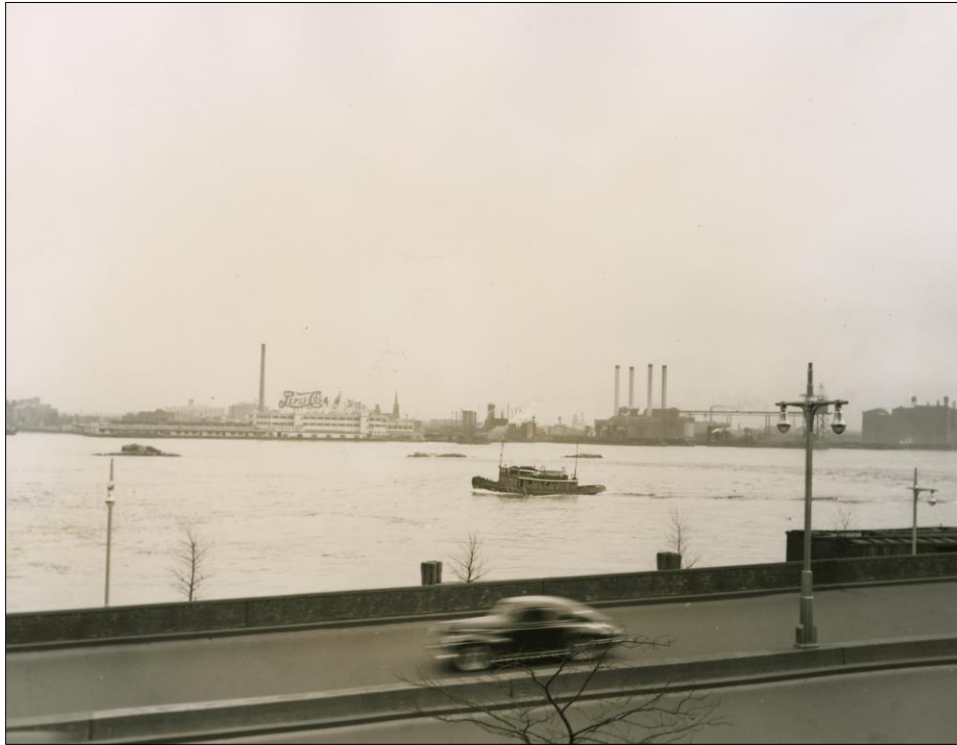
Pepsi-Cola Sign as it appeared in its original form, undated. Photo: Courtesy of PepsiCo
