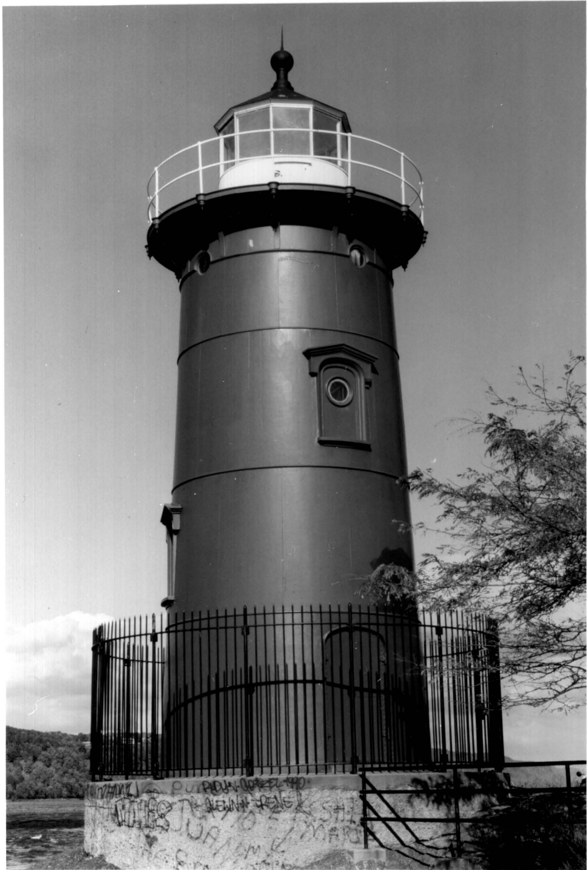
Jeffrey's Hook Lighthouse, Fort Washington Park, Manhattan. Photo credit: Betsy Bradley
