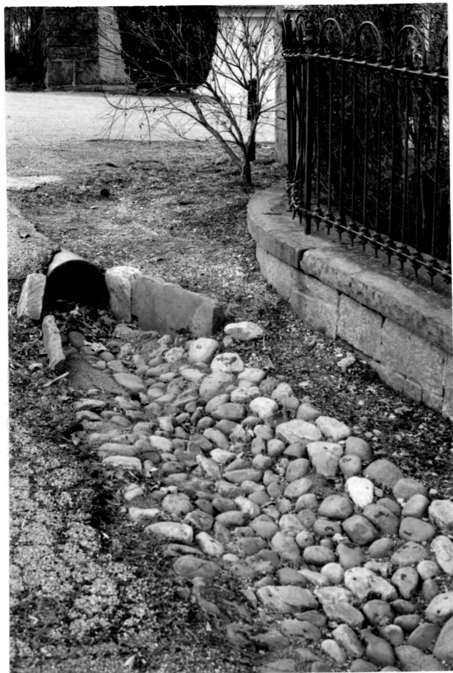
Sycamore Avenue, street drainage system
