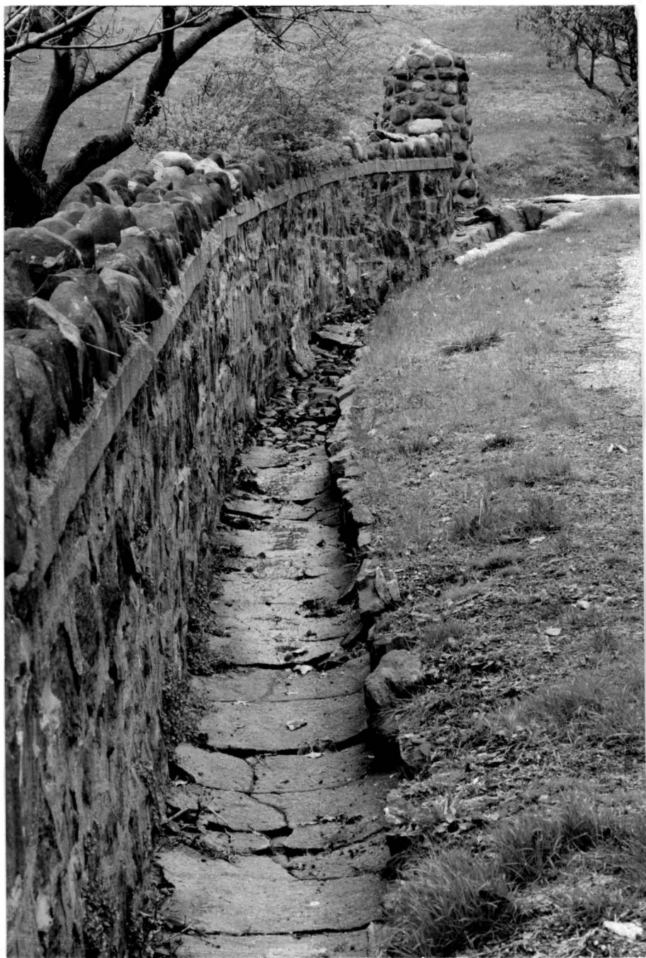
Sycamore Avenue, street drainage system
