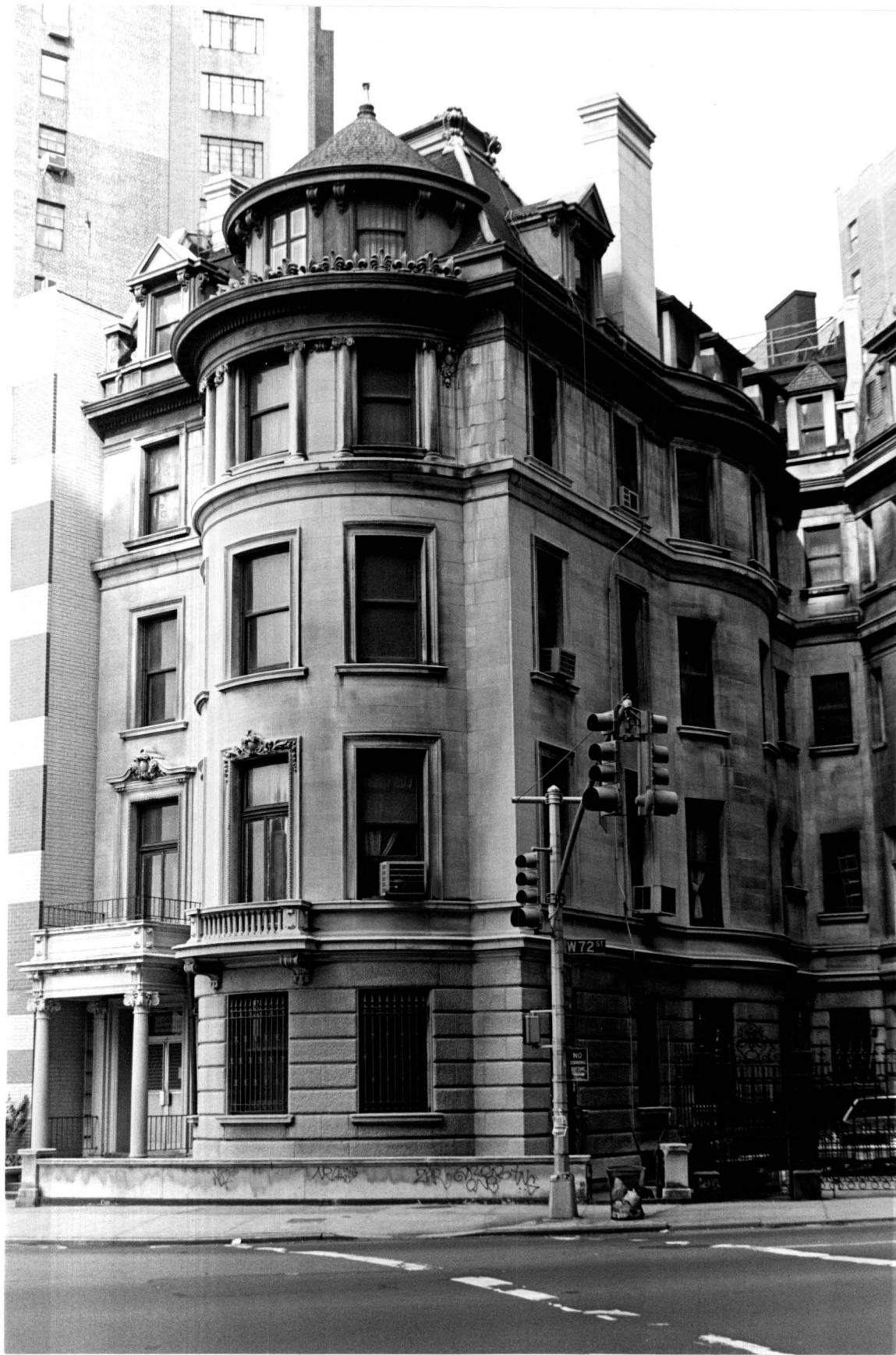
The Prentiss Residence, View with Side Elevation. Photo Credit: Carl Forster.
