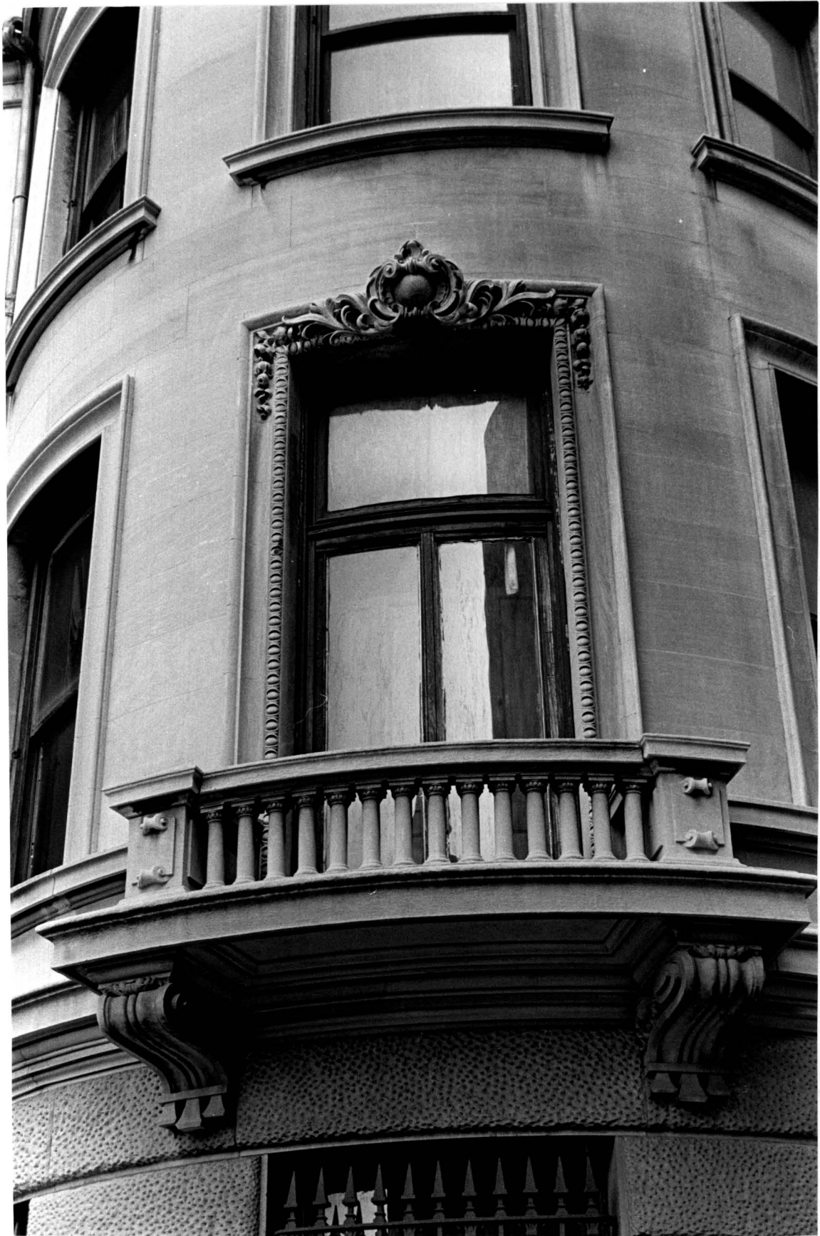
The Prentiss Residence, Detail of Window. Photo Credit: Carl Forster.
