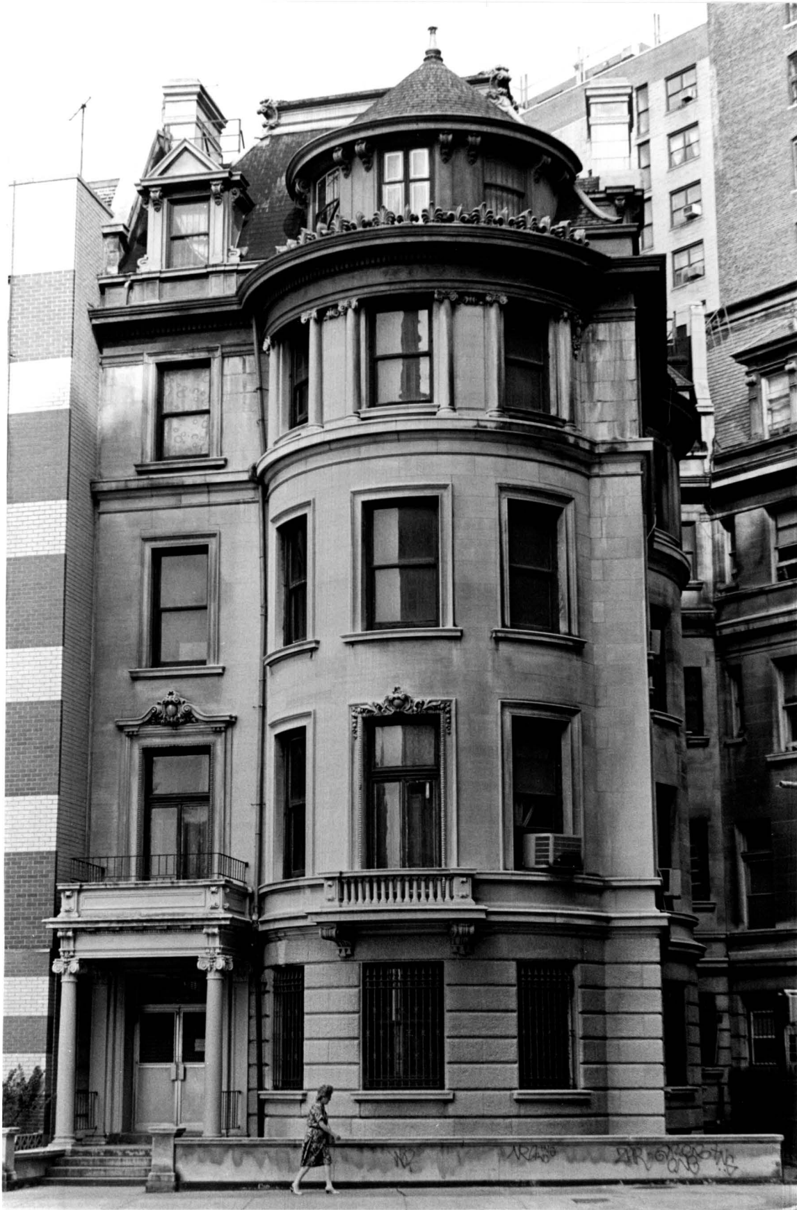
The Prentiss Residence, 1 Riverside Drive. C.P.H. Gilbert, 1899-1901. Photo Credit: Carl Forster.
