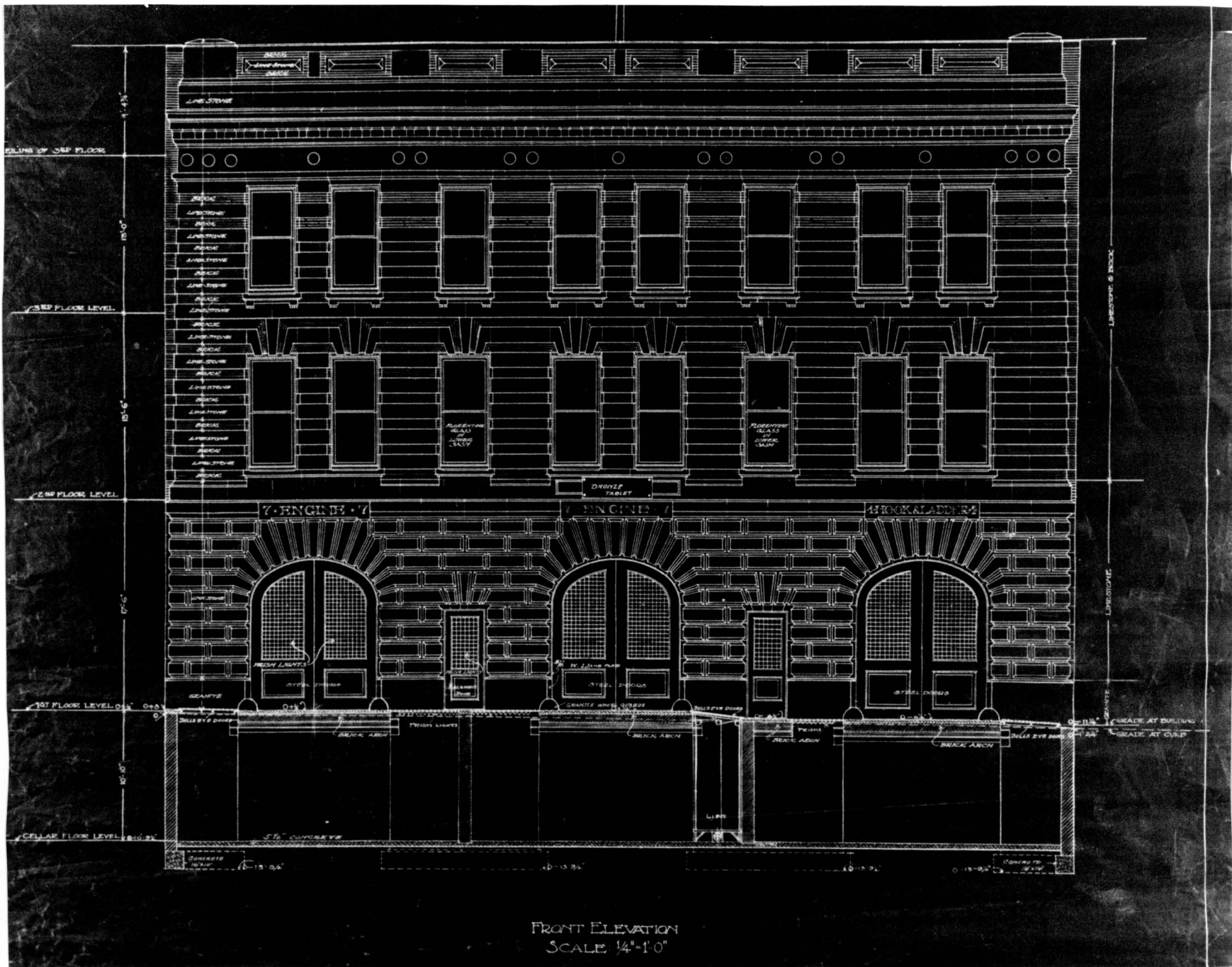
Plate 1. Trowbridge & Livingston, Blueprint drawing for the Front Elevation of Engine Company No. 7/Hook & Ladder No. 1, 1904. Buildings Division, NYC Fire Department.
