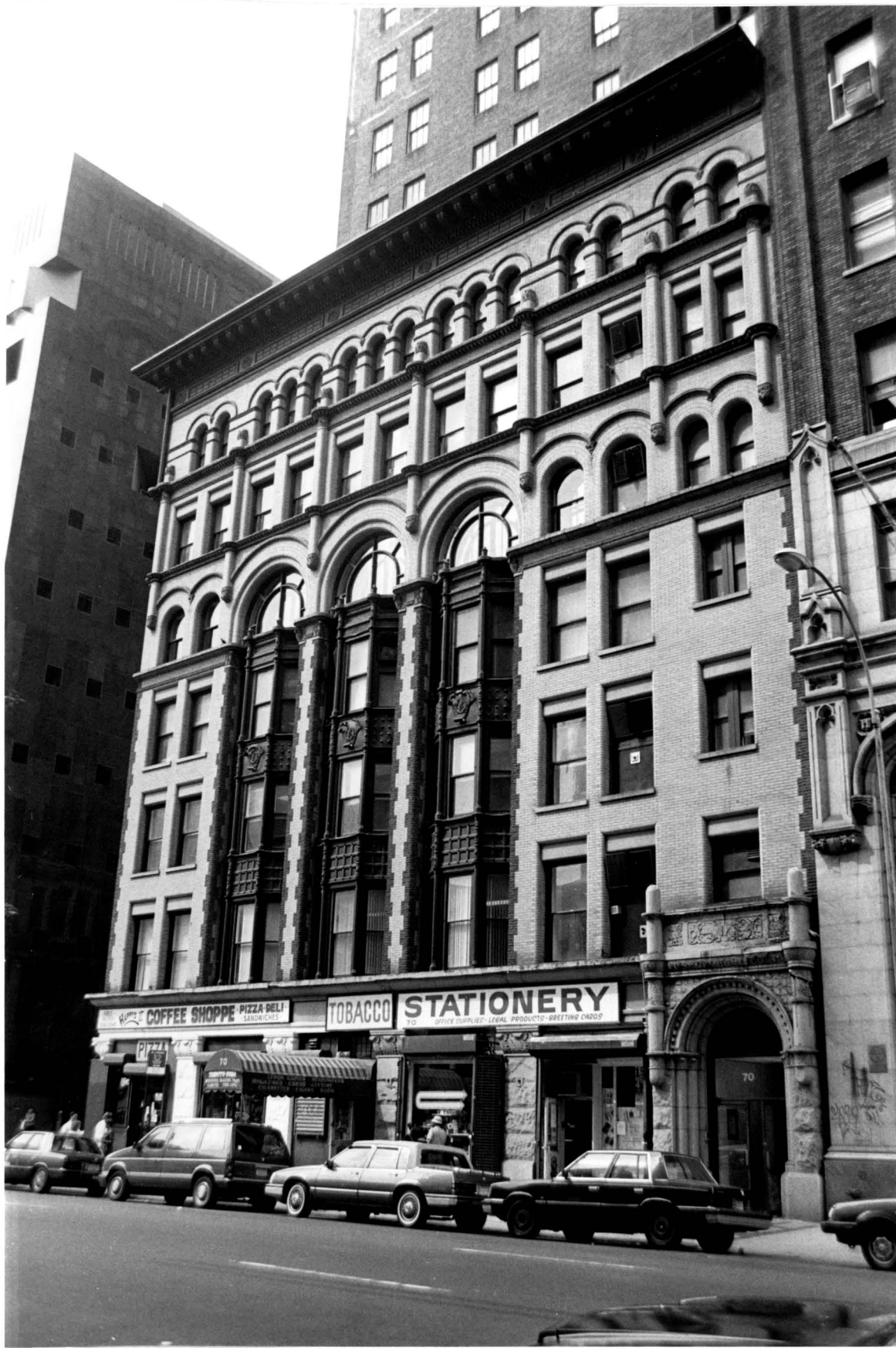
Ahrens Building, 70-76 Lafayette Street Lafayette Street facade
