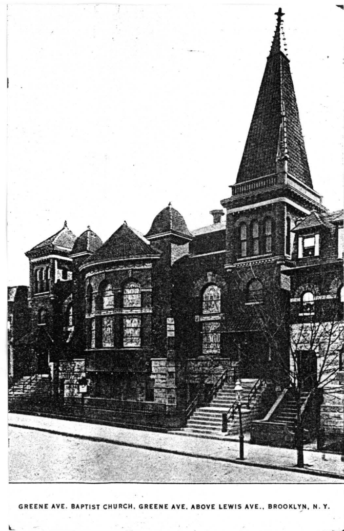
Fig. 3 Greene Avenue Baptist Church, early twentieth-century postcard view in the LPC files
