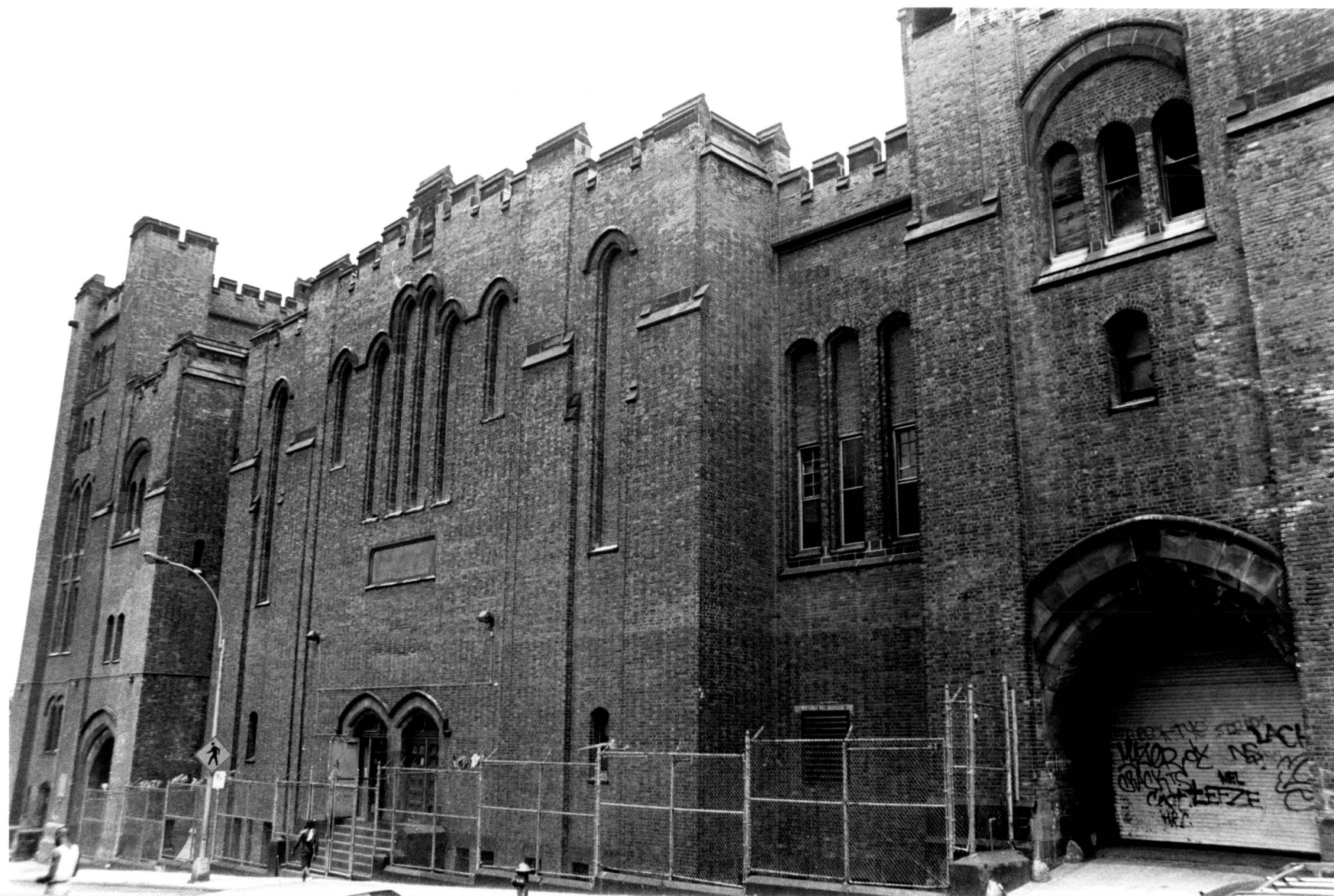
Fig. K. Second Battery Armory, 166th Street facade
