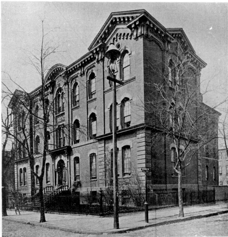
Fig. 9 Public School 24 Demolished
