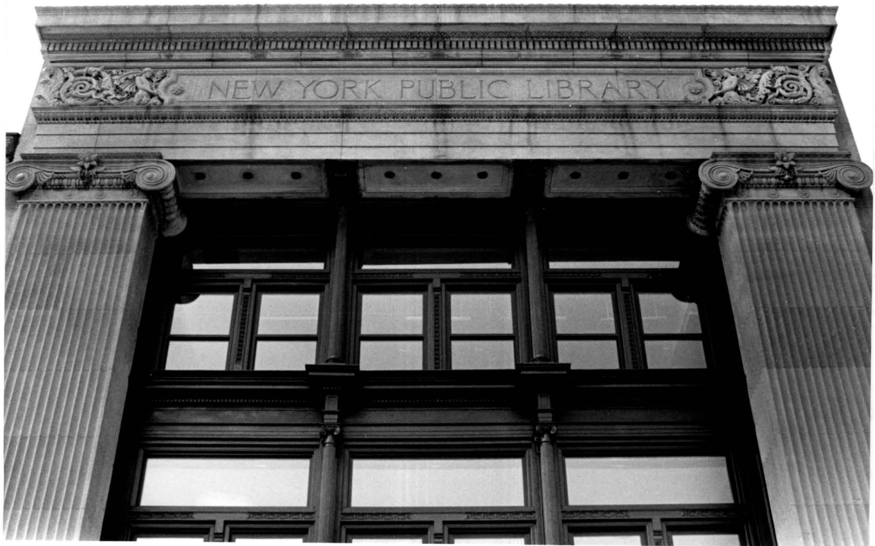
Fig. 3 Detail: Ionic capitals supporting entablature
