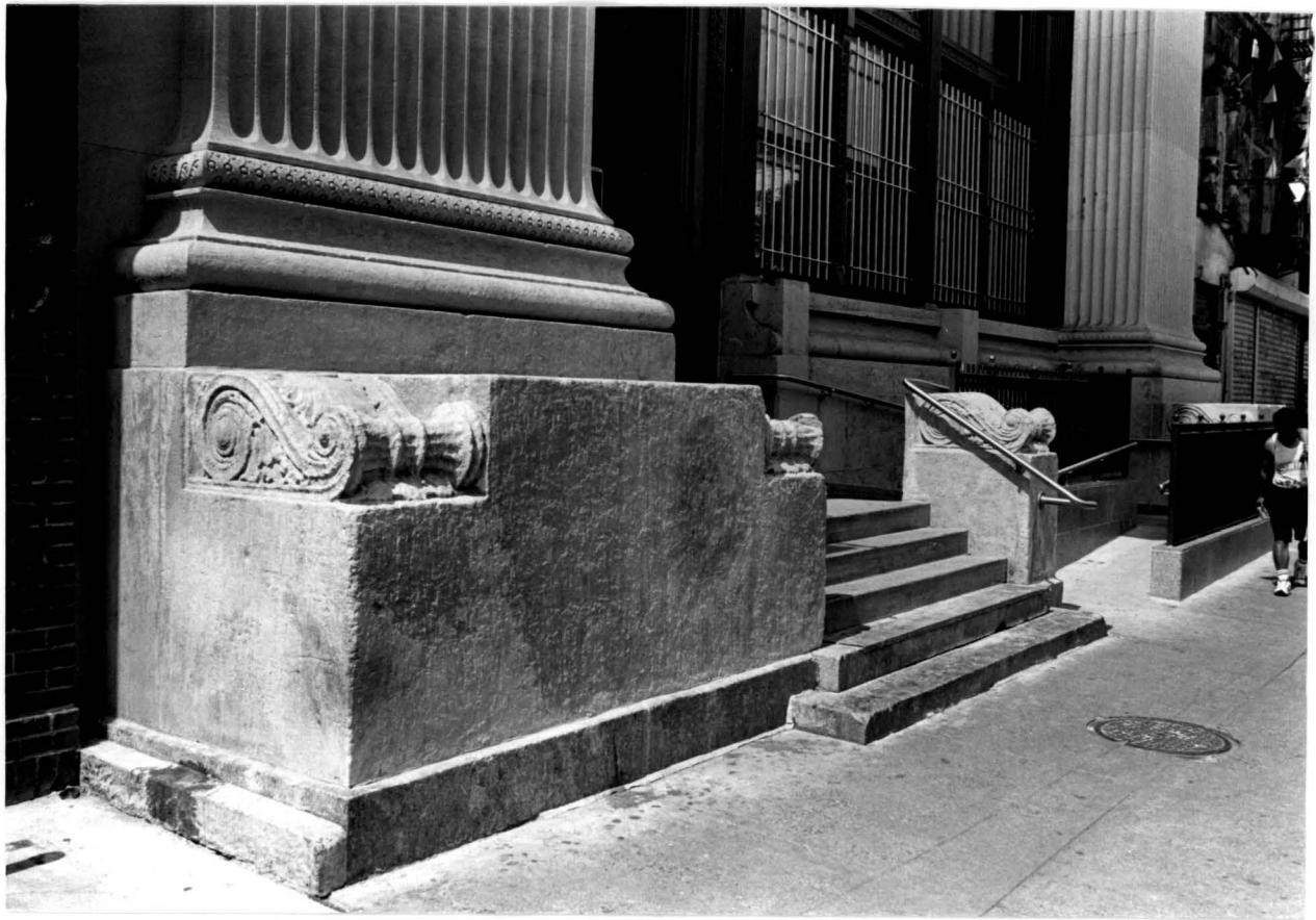
Fig. 2 Detail: Limestone pier on granite base
