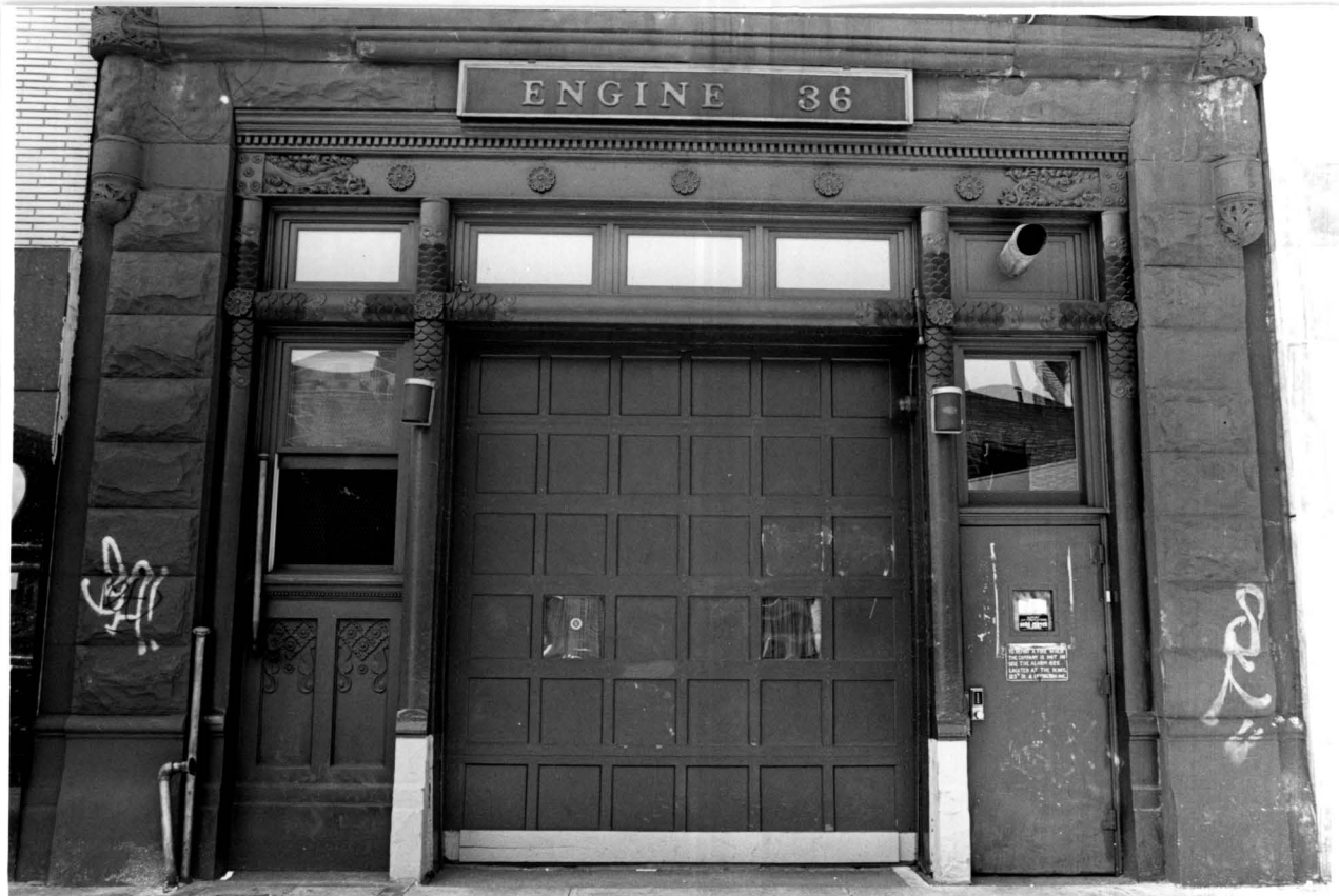
Fire Hook & Ladder Company No. 14 (now Fire Engine Company No. 36) View of base Photo: Carl Forster
