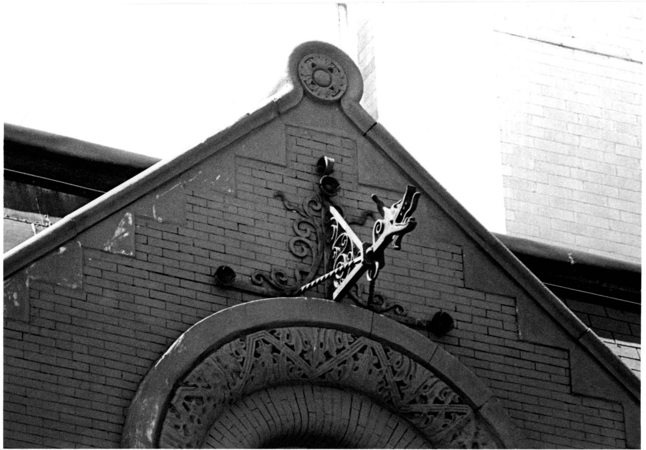
Fire Hook & Ladder Company No. 14 (now Fire Engine Company No. 36) Detail of wrought-iron jib used for hauling hay Photo: Carl Forster
