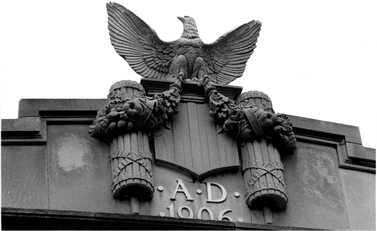
Fire Engine Company No. 84 and Hook & Ladder Company No. 34 Detail of cornice Photo: Carl Forster
