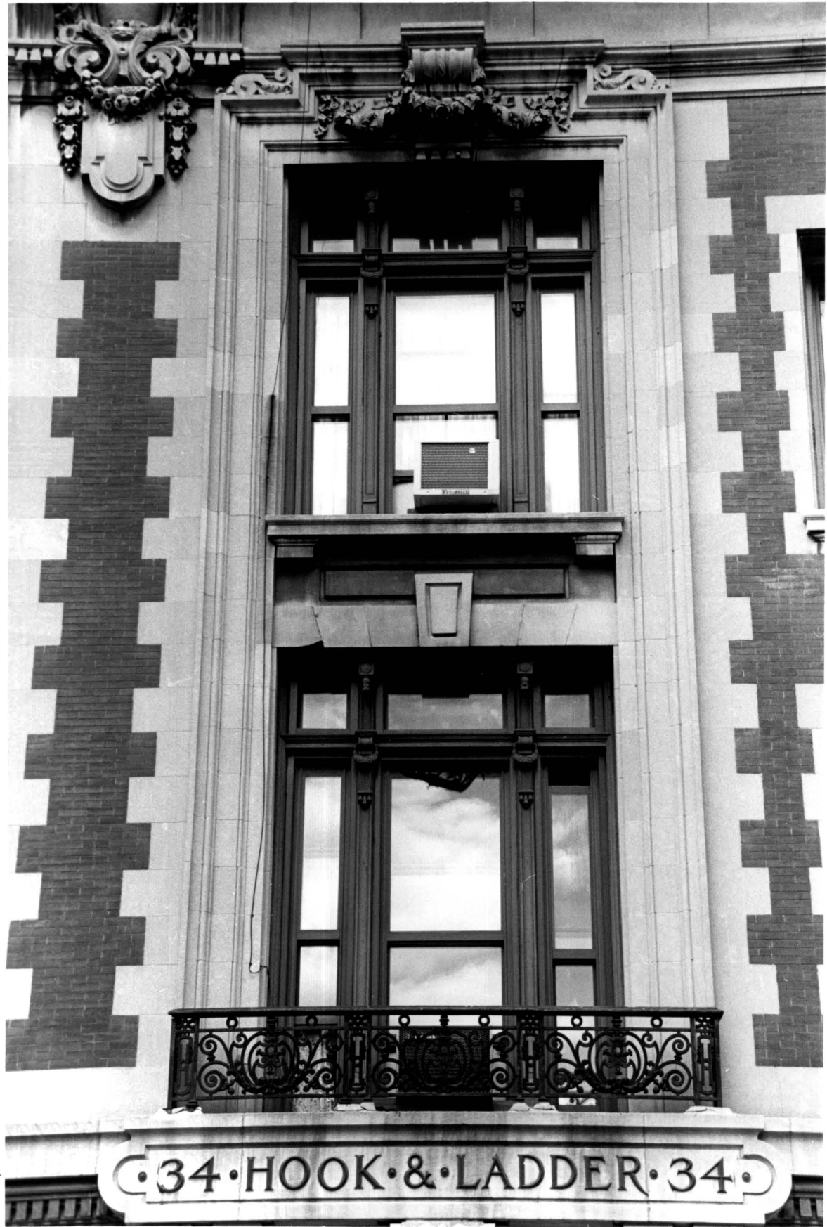
Fire Engine Company No. 84 and Hook & Ladder Company No. 34 Detail of window bay Photo: Carl Forster
