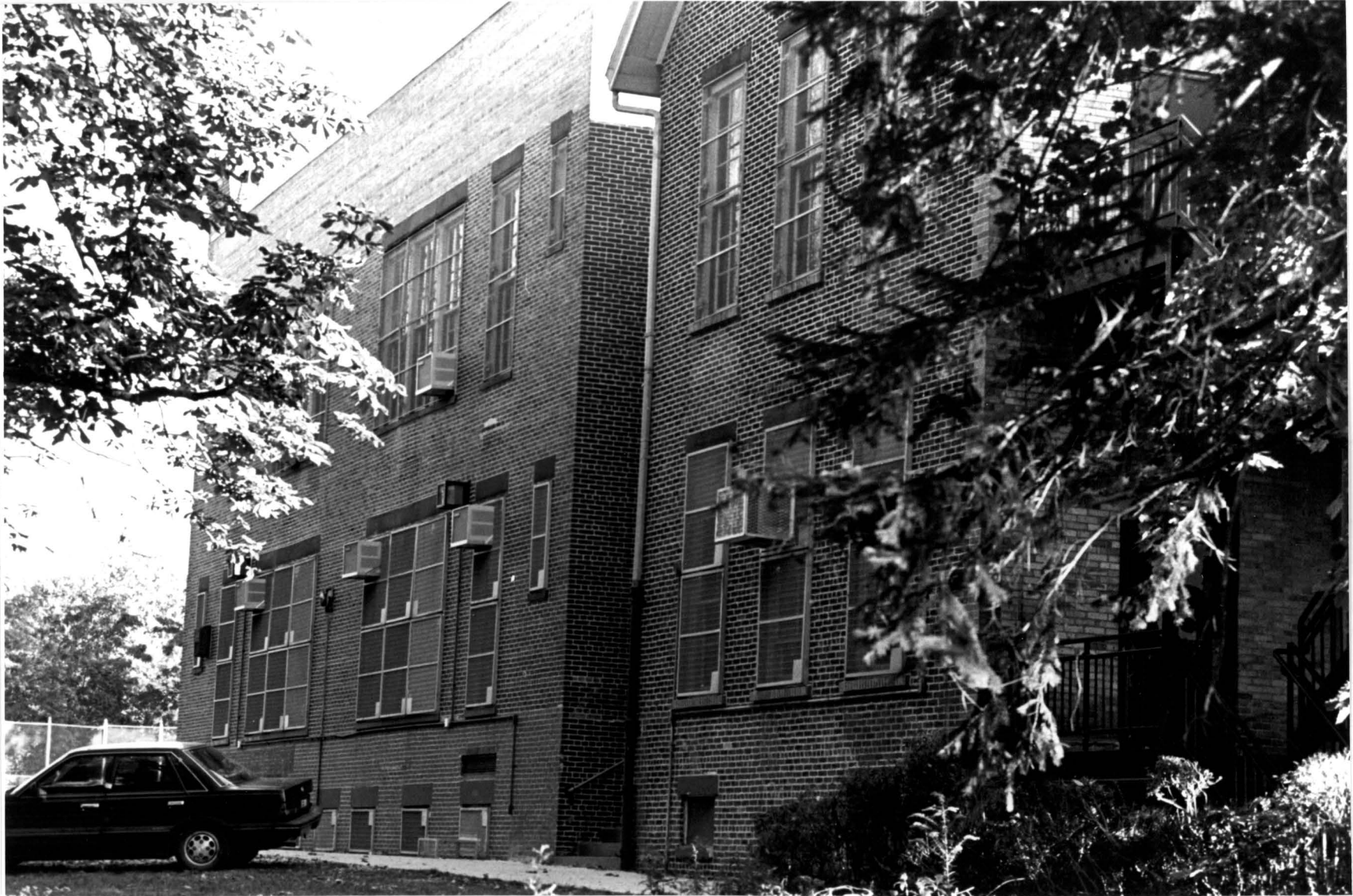
Westfield Township District School No. 7 (later Public School No. 4), 4210-4212 Arthur Kill Road, Charleston, Staten Island. North facade, original wing on the right, addition on the left.
