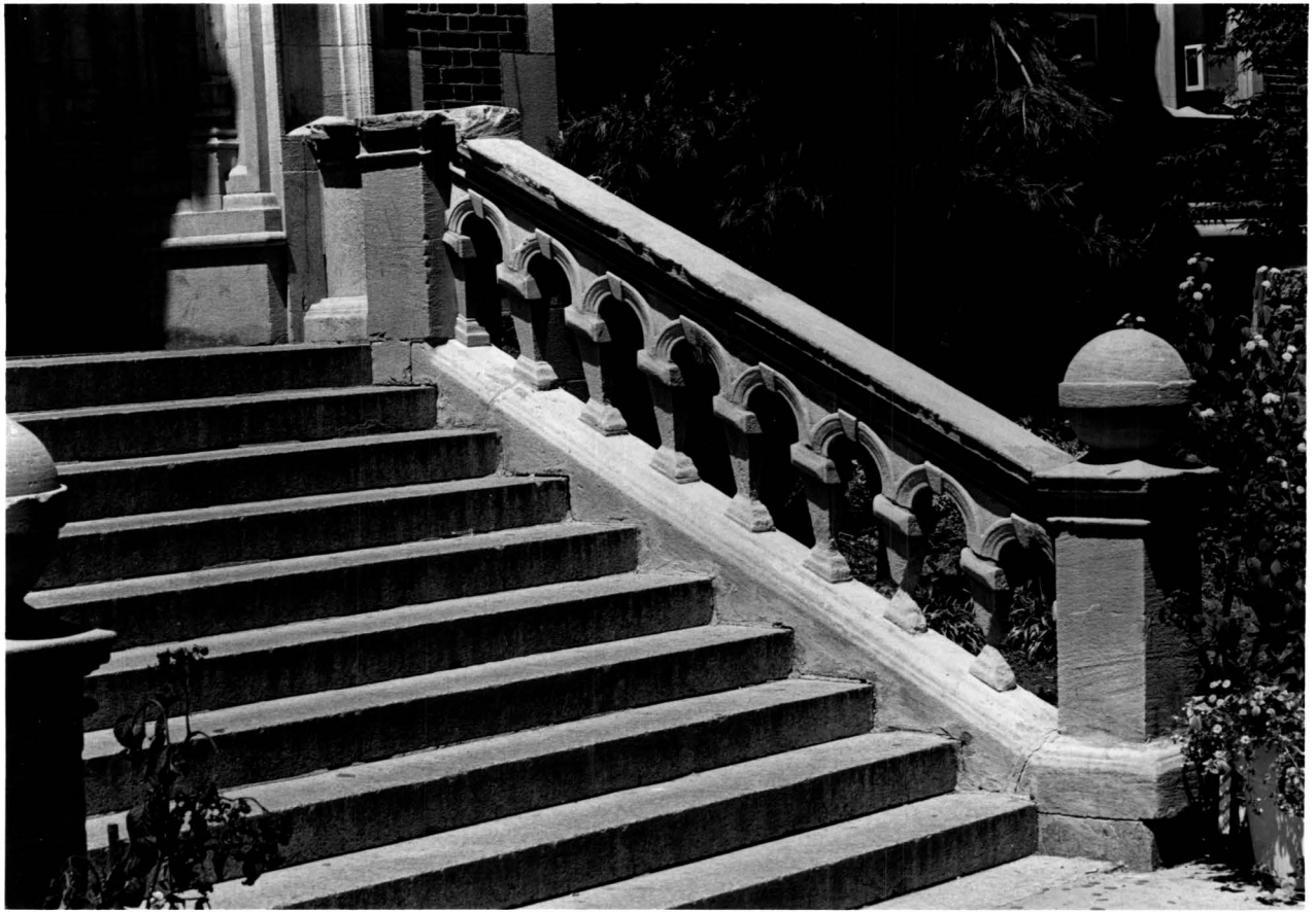
Messiah Home for Children Main entrance stairway
