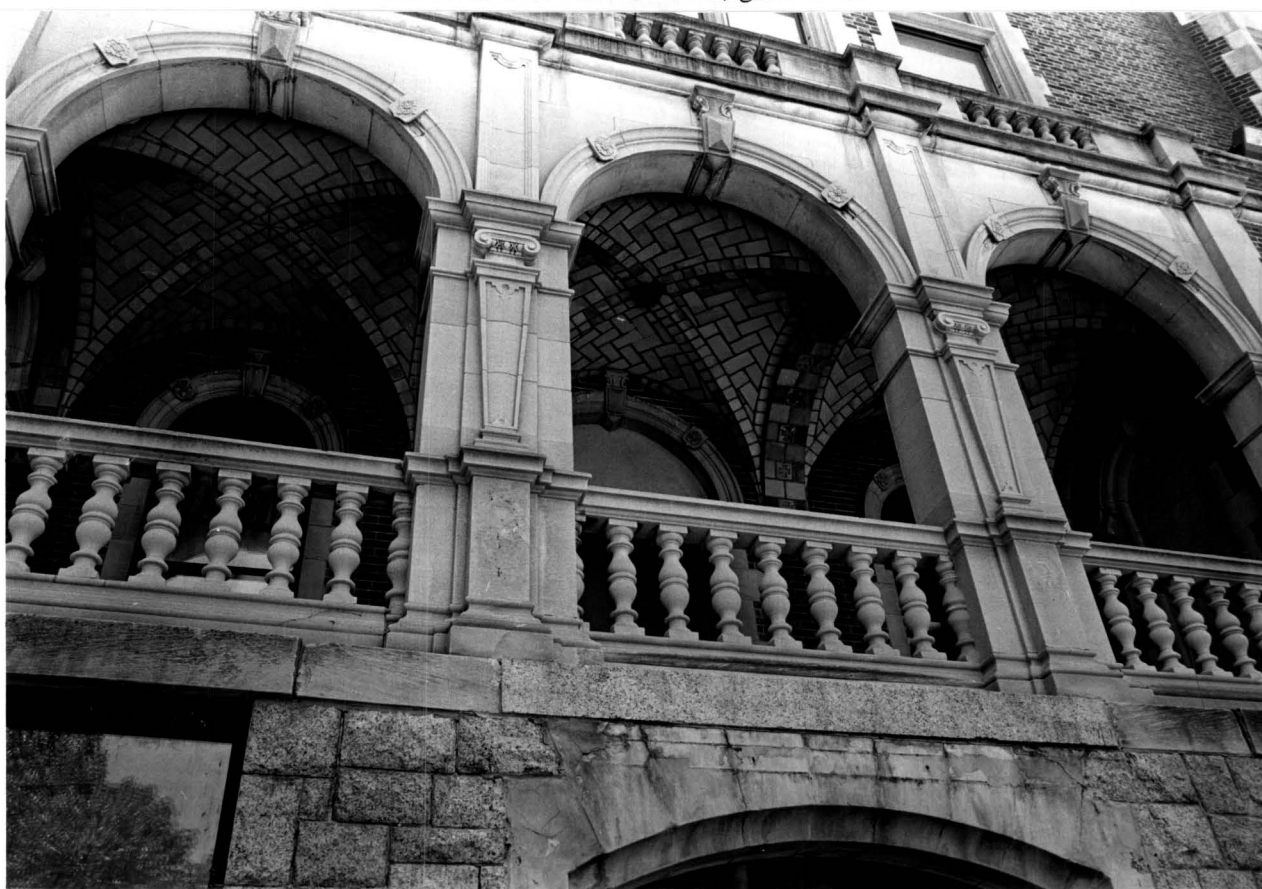
Messiah Home for Children West Tremont Avenue elevation, porch detail
