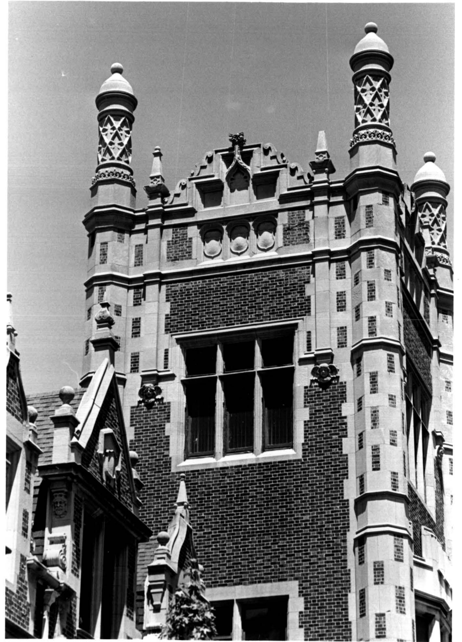
Messiah Home for Children Entrance Tower detail Photo: Carl Forster
