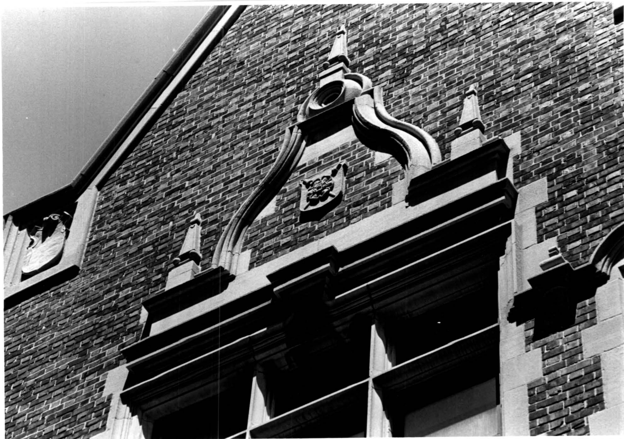
Messiah Home for Children West Tremont Avenue elevation, gable detail
