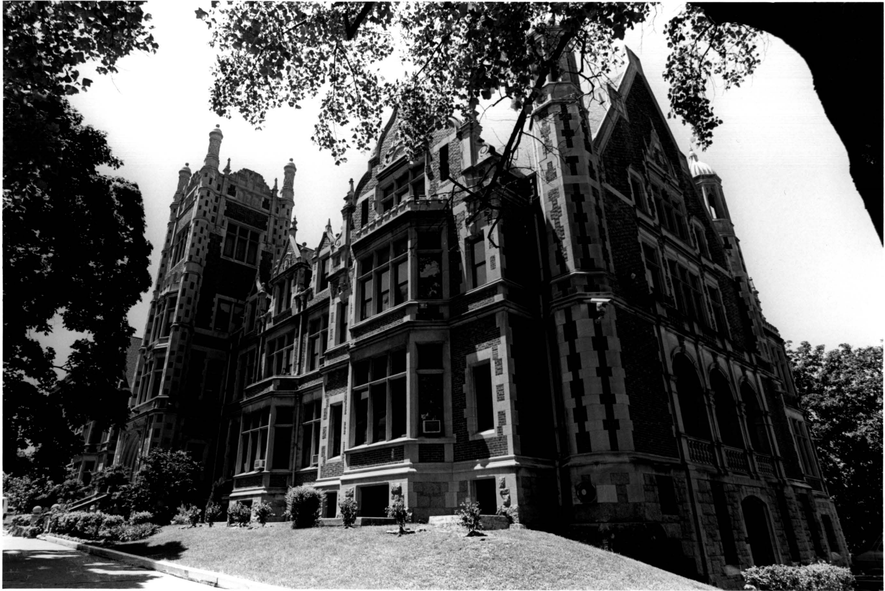
Messiah Home for Children, 1771-1777 Andrews Avenue South, The Bronx Andrews Avenue South and West Tremont Avenue elevations Photo: Carl Forster
