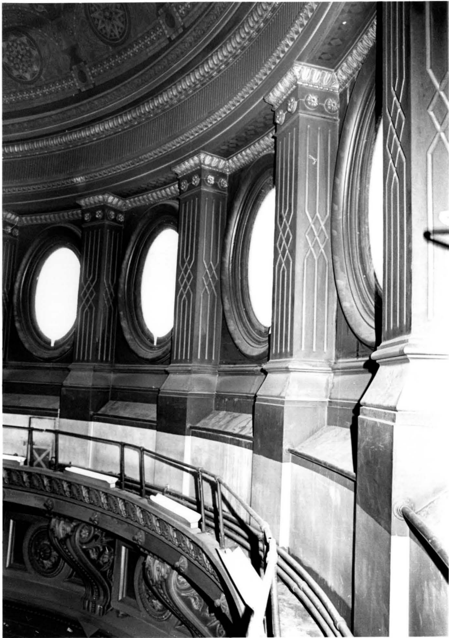
Williamsburgh Savings Bank (Broadway) Details of the cast iron drum and gallery
