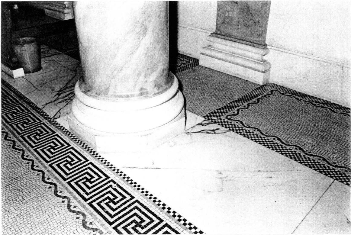
16. Mosaic Floor, Waiting Room
