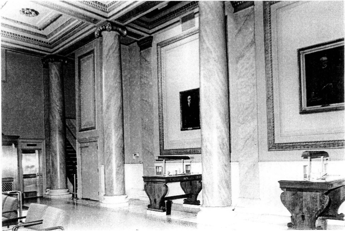
13. Waiting Room, Elevator Shaft inserted in South Aisle
