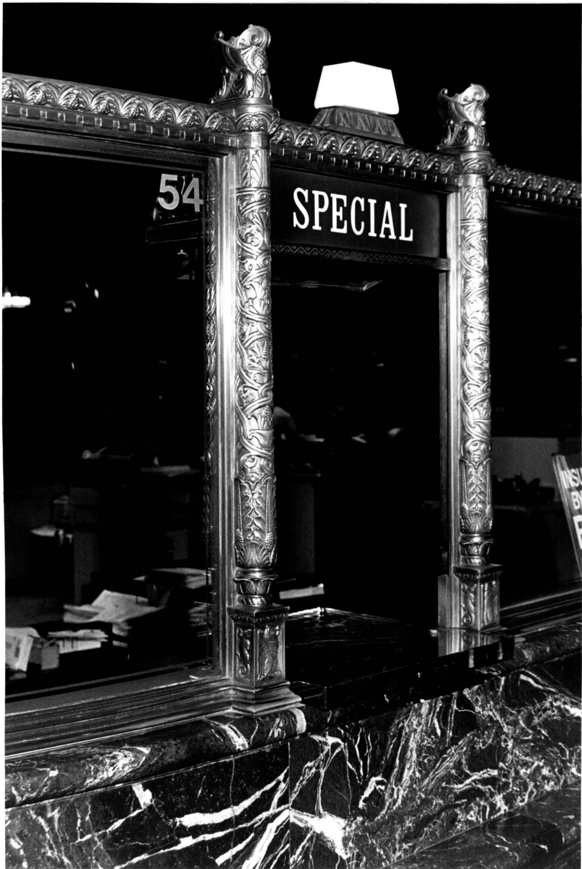
Bowery Savings Bank Building - Banking Room Detail of tellers' counter
