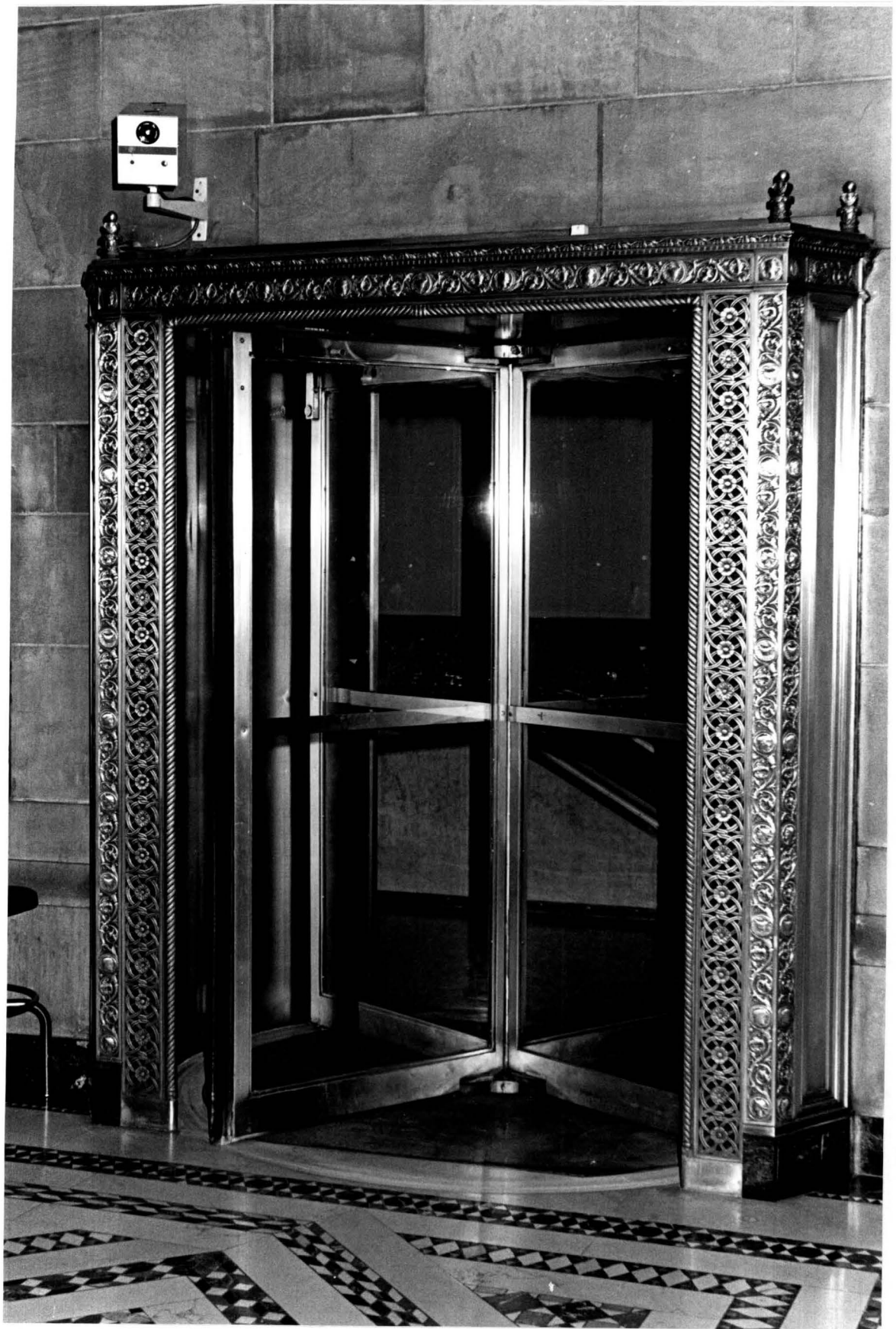
Bowery Savings Bank Building - Banking Room Revolving door housing at northwest corner to office building vestibule
