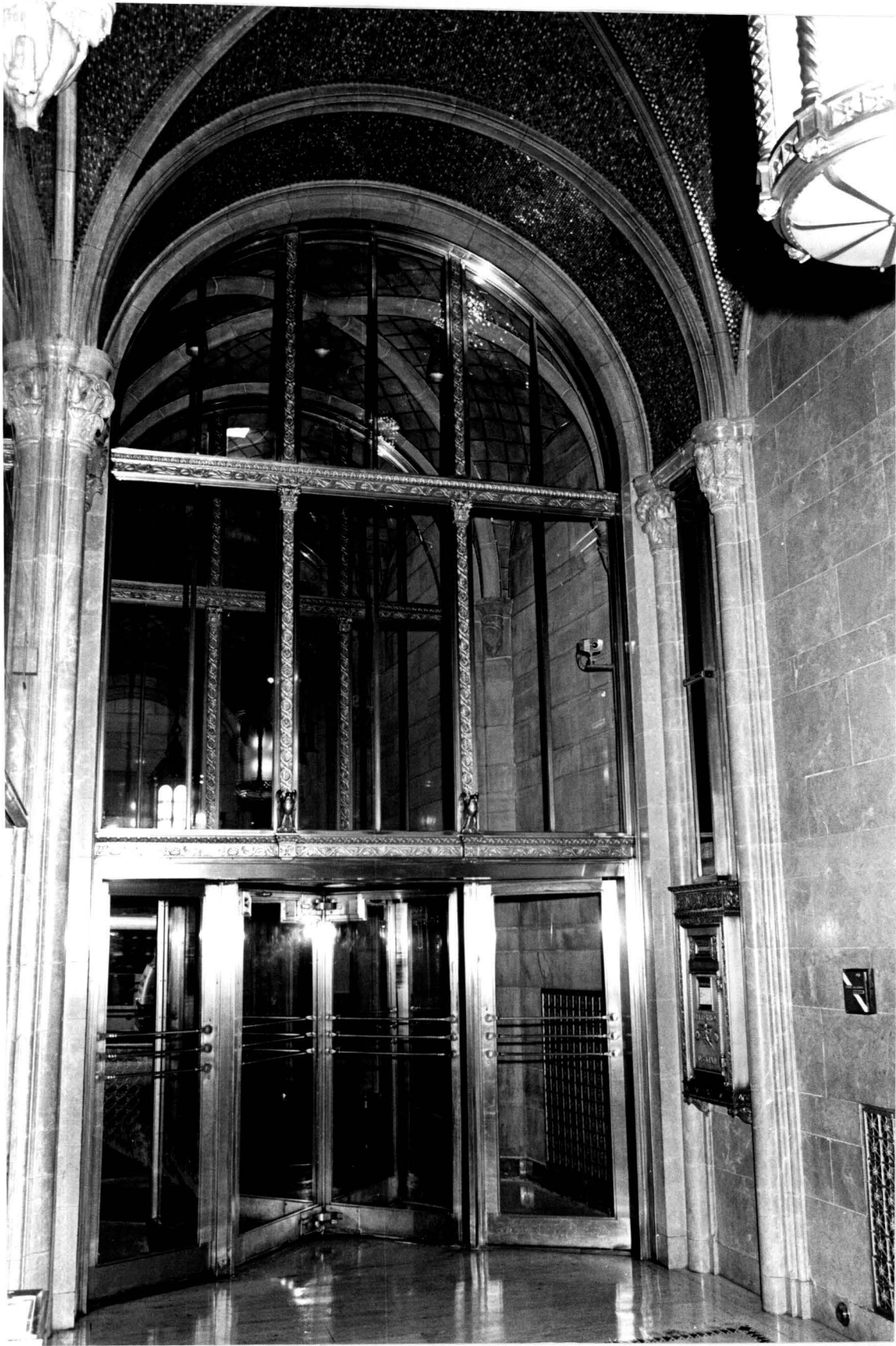
Bowery Savings Bank Building - Elevator Lobby Detail of doorway to entrance vestibule
