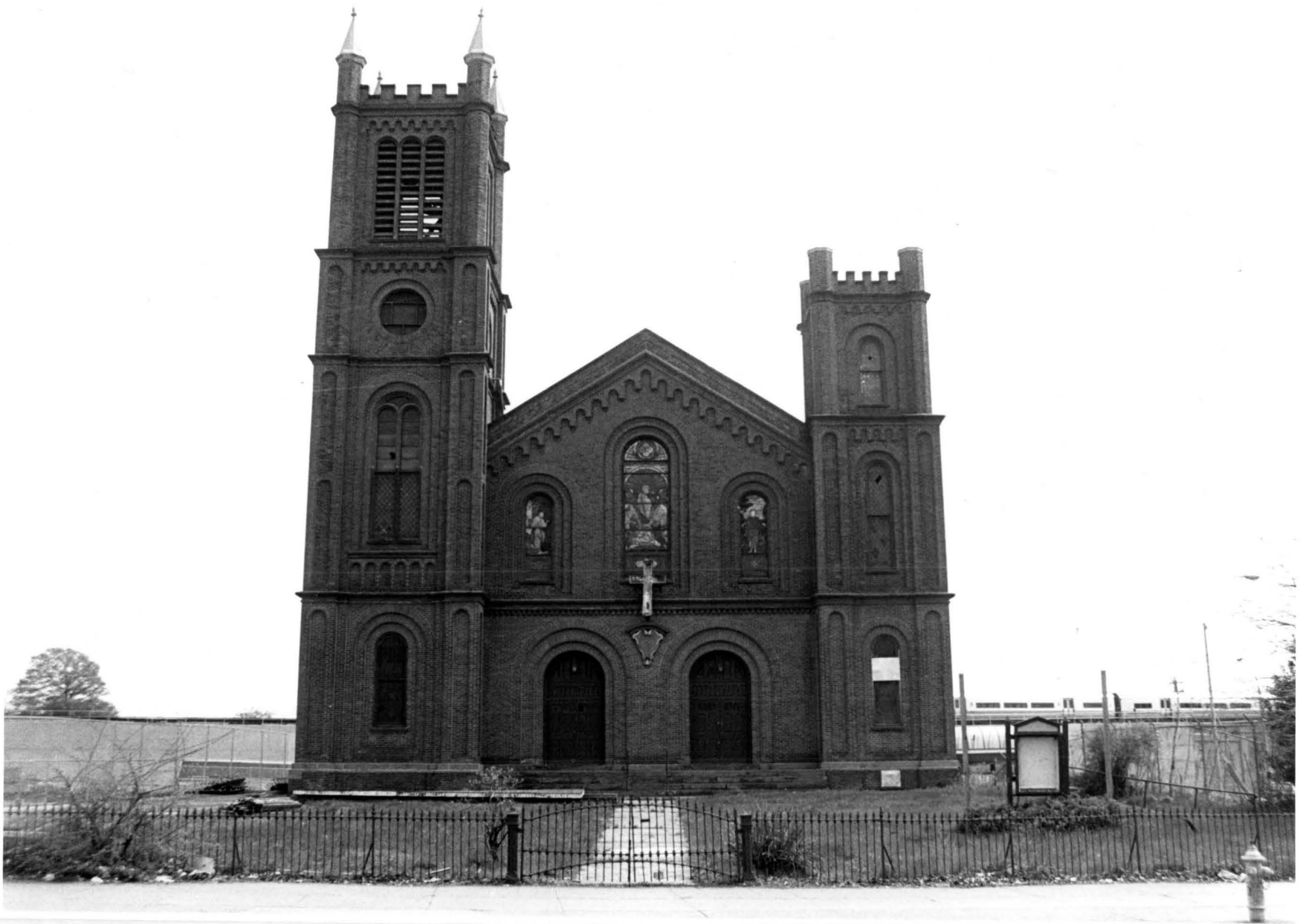
First Reformed Church of Jamaica Jamaica Avenue facade
