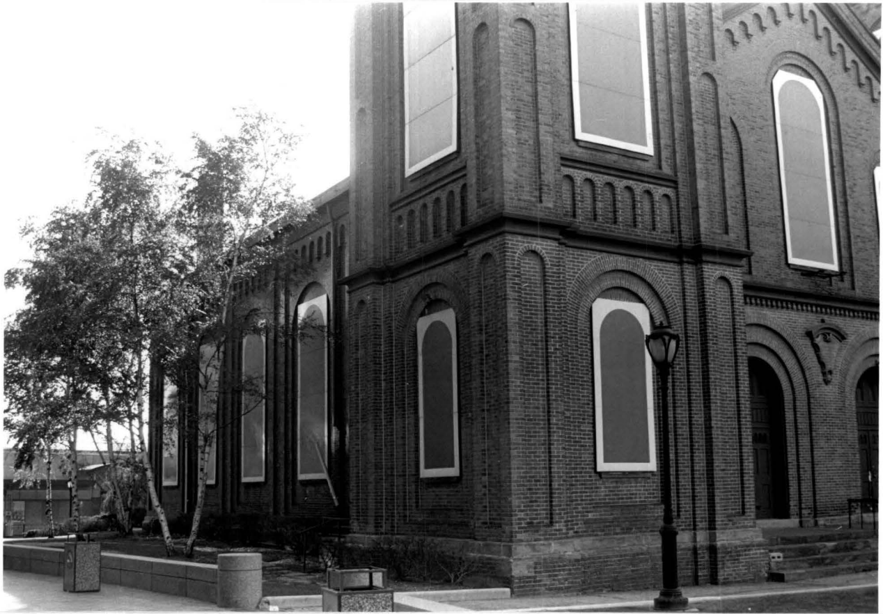
East elevation, showing the base of the east tower
