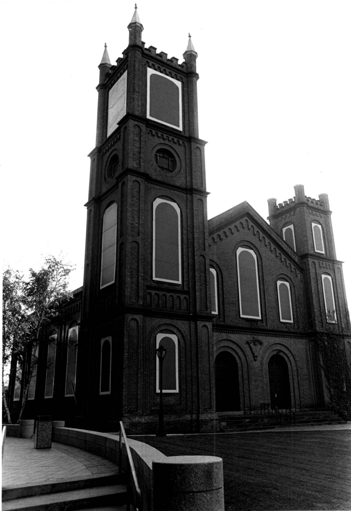
First Reformed Church of Jamaica, 153-10 Jamaica Avenue, Queens. Jamaica Avenue facade from the northeast.
