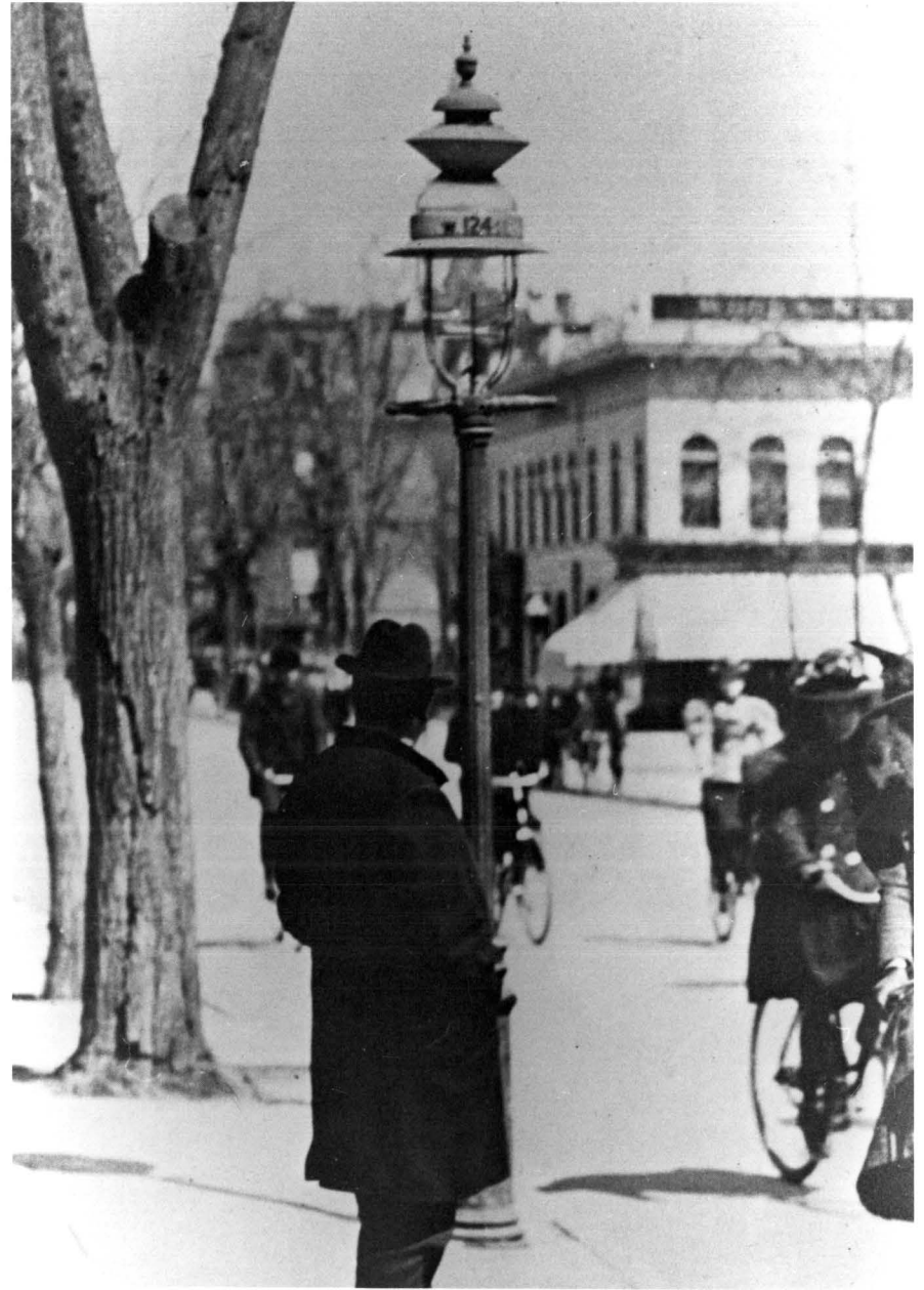
fig. 5. Detail of second type of gas luminaire (Pennsylvania Globe Gas Light Co. "Manhattan" type). Theodore James Jr., Fifth Avenue , p. 190.
