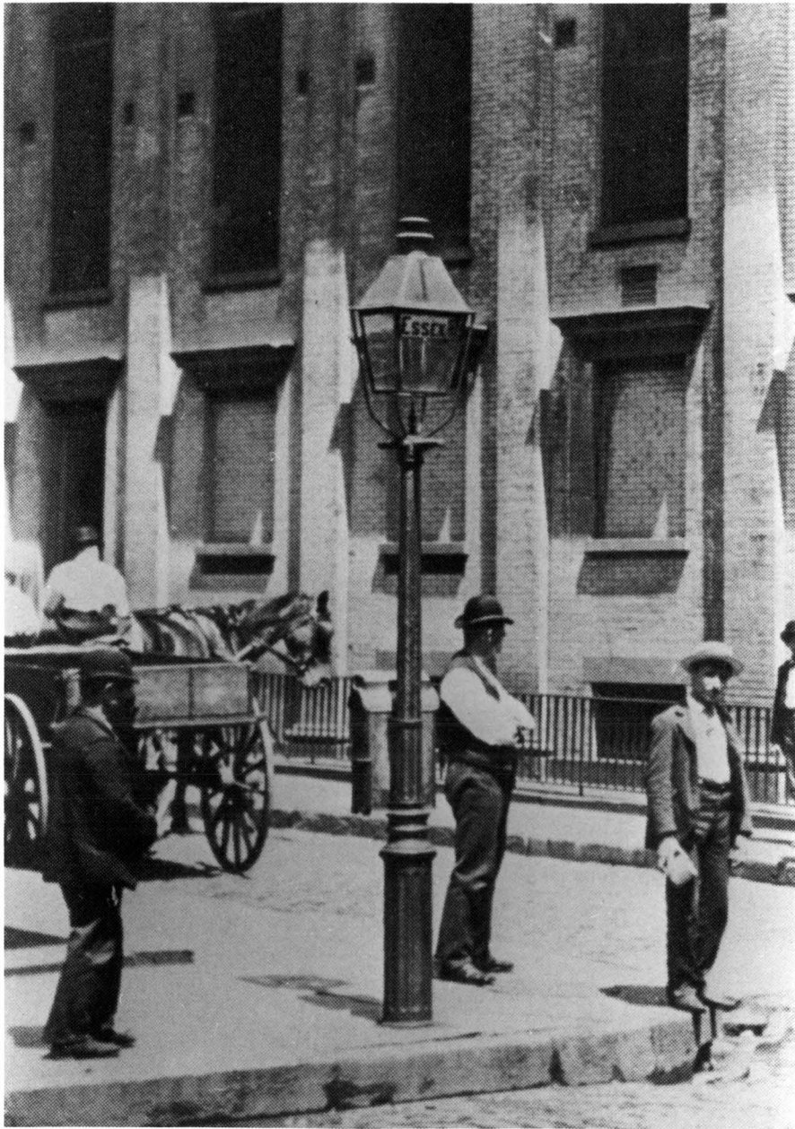
fig. 4. Standard gas lamppost with early luminaire (Pennsylvania Globe Gas Light Co., "New York Corporation" type). Black, pl. 79, p. 90.
