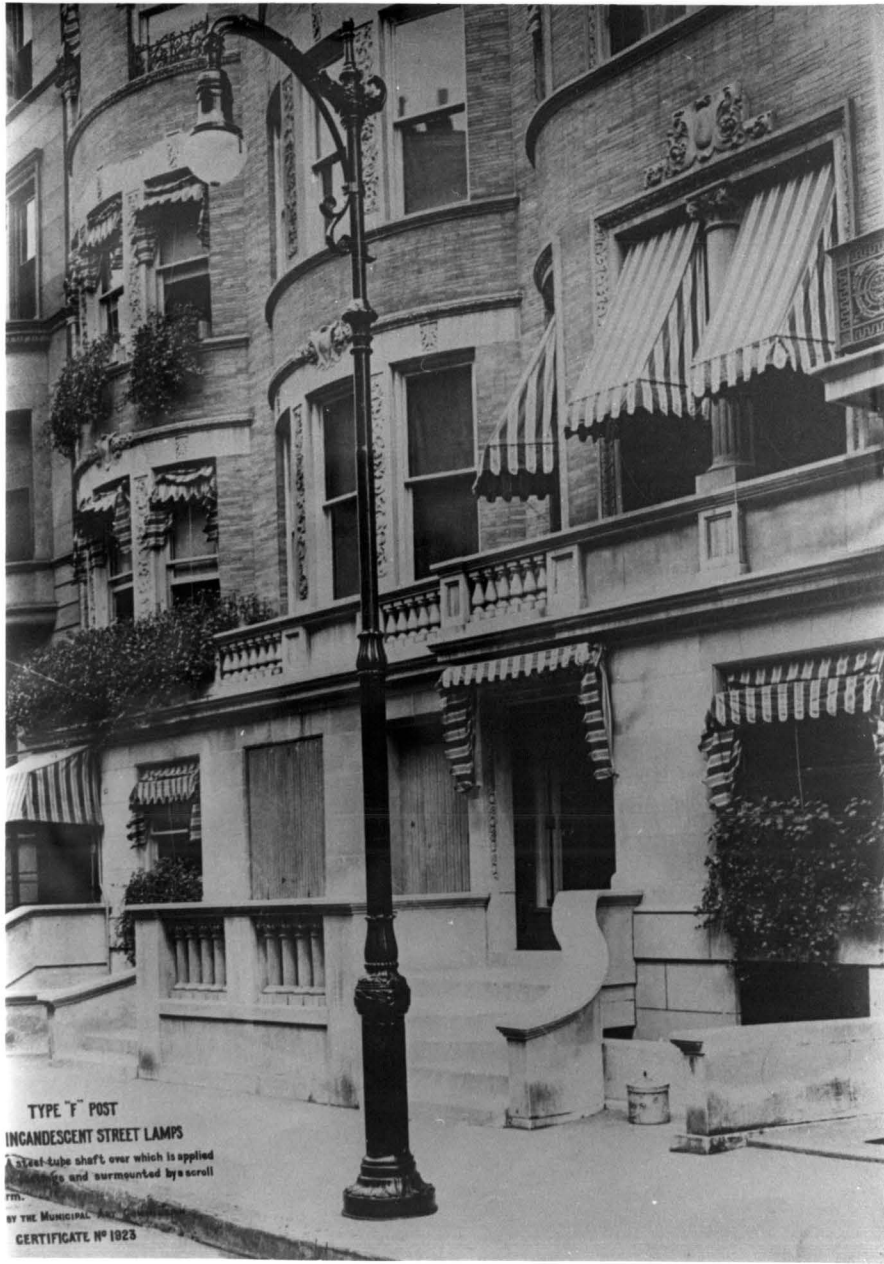
fig. 24. Type F. Known originally as a "reverse scroll bracket," this type was an alternative to the bishop's crook, and was most commonly found on residential side streets. Art Commission of the City of New York.
