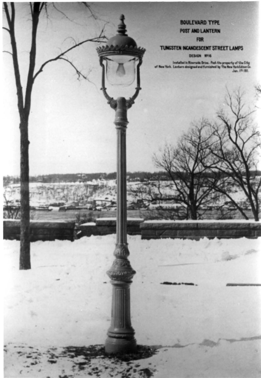
fig. 16. Boulevard, or Type C, short post, probably originally designed for gas and retrofitted for early incandescent lamps. Used on boulevards, such as Broadway, and park-like drives, such as Riverside Drive. Art Commission of the City of New York.
