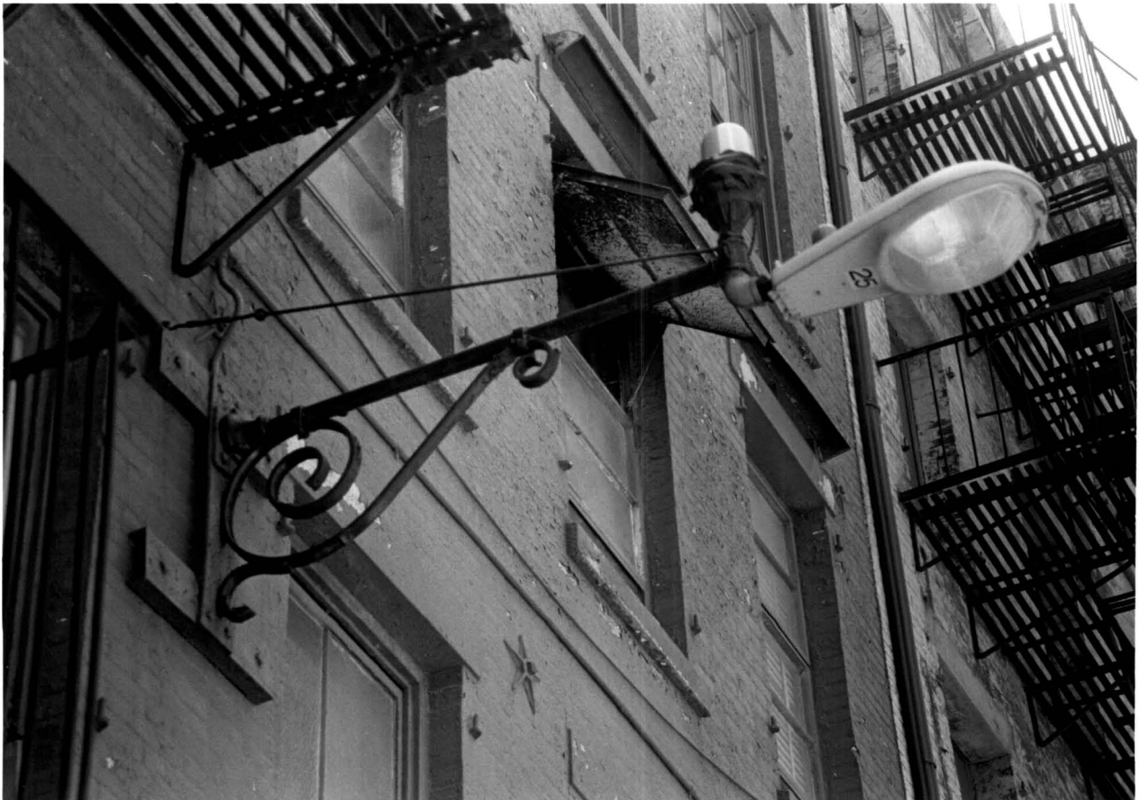
fig. 34. Special Combination Bracket. Includes a light identifying the presence of a nearby fire alarm box. Landmarks Preservation Commission.
