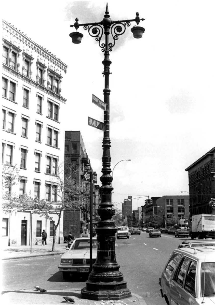
fig. 31. The last New York Electric Co. Type 6. Landmarks Preservation Commission.
