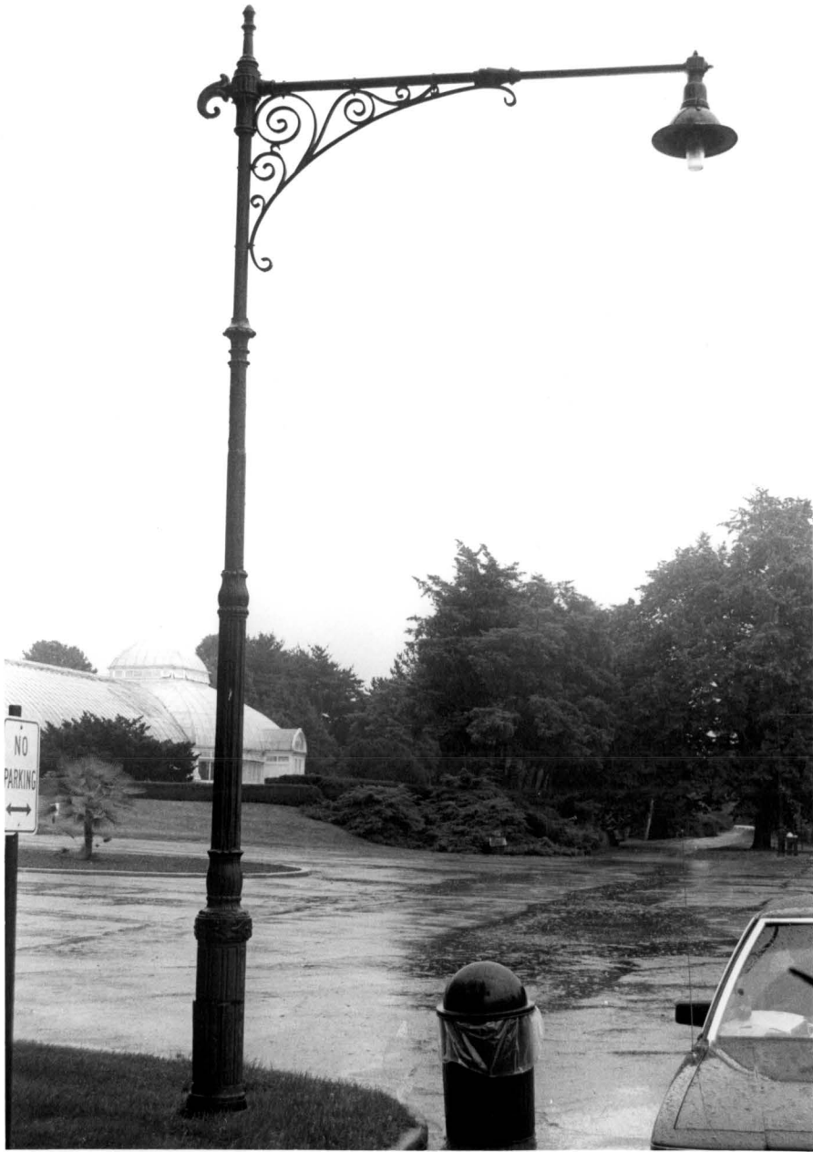
fig. 22. Type G. The other mast-arm type. The base is modelled after Henry Bacon's short park post of 1911. This design was frequently, but not exclusively, used on park drives. Landmarks Preservation Commission.
