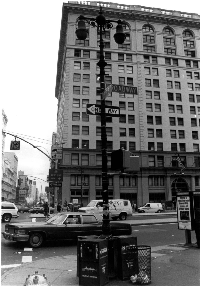
fig. 26. Type 1 Twin. An early hybrid type, featuring a Type 1BC post and a Type 3 Twin top. Landmarks Preservation Commission.
