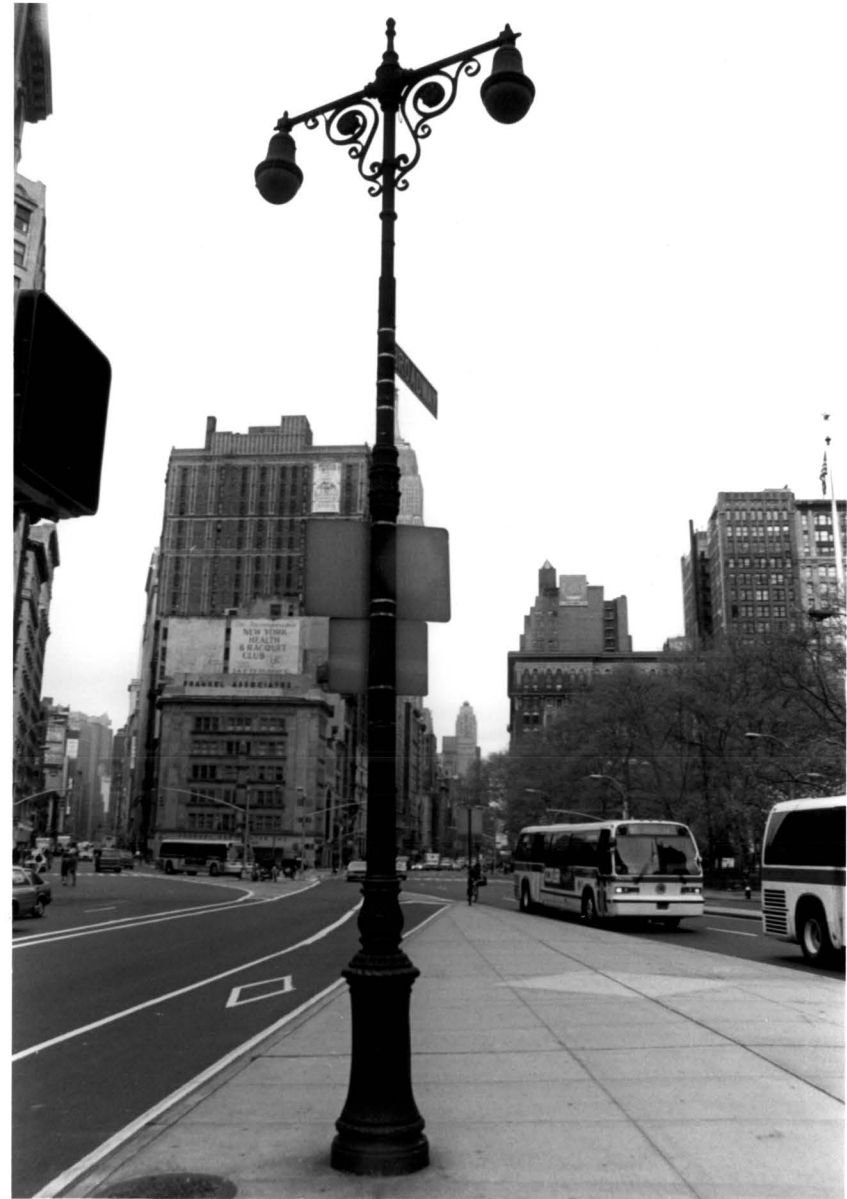
fig. 27. Type 24 Twin. A descendent of the old Fifth Avenue twin post, this design served as the model for the reproduction posts around Bryant Park. Landmarks Preservation Commission.
