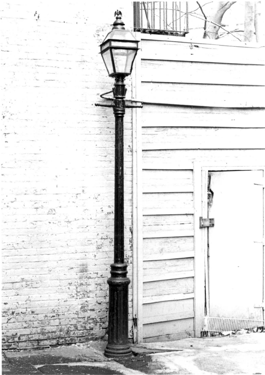
fig. 35. Gas post. One of two remaining. This type was used throughout the city from the mid-19th century to the end of the gas light era. Landmarks Preservation Commission.
