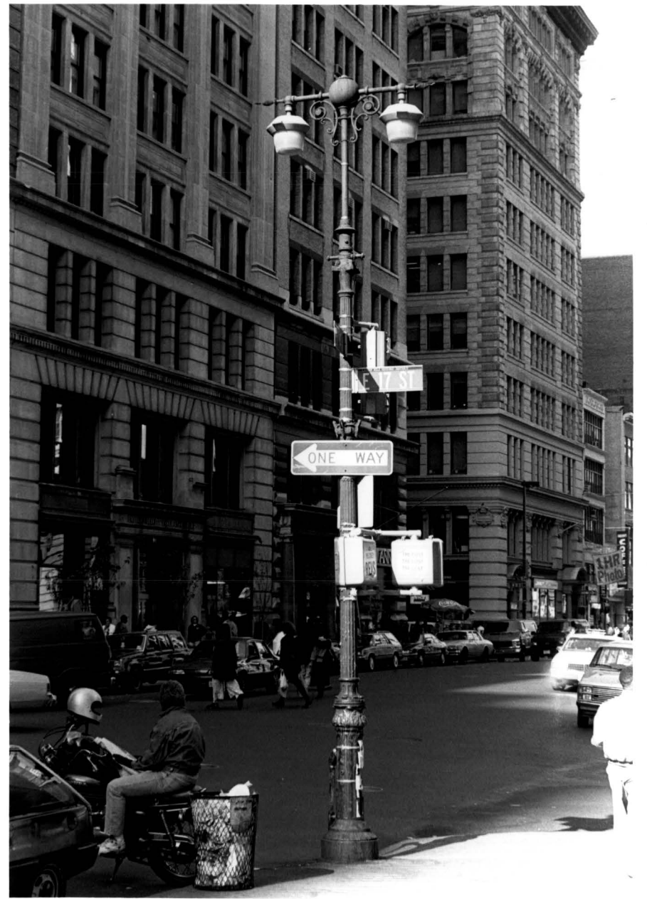
fig. 25. Type 3 Twin. Old Fifth Avenue twin post. This post is the last remaining from the 1892 installation on Fifth Avenue. Photograph taken just prior to the post's recent restoration. Landmarks Preservation Commission.
