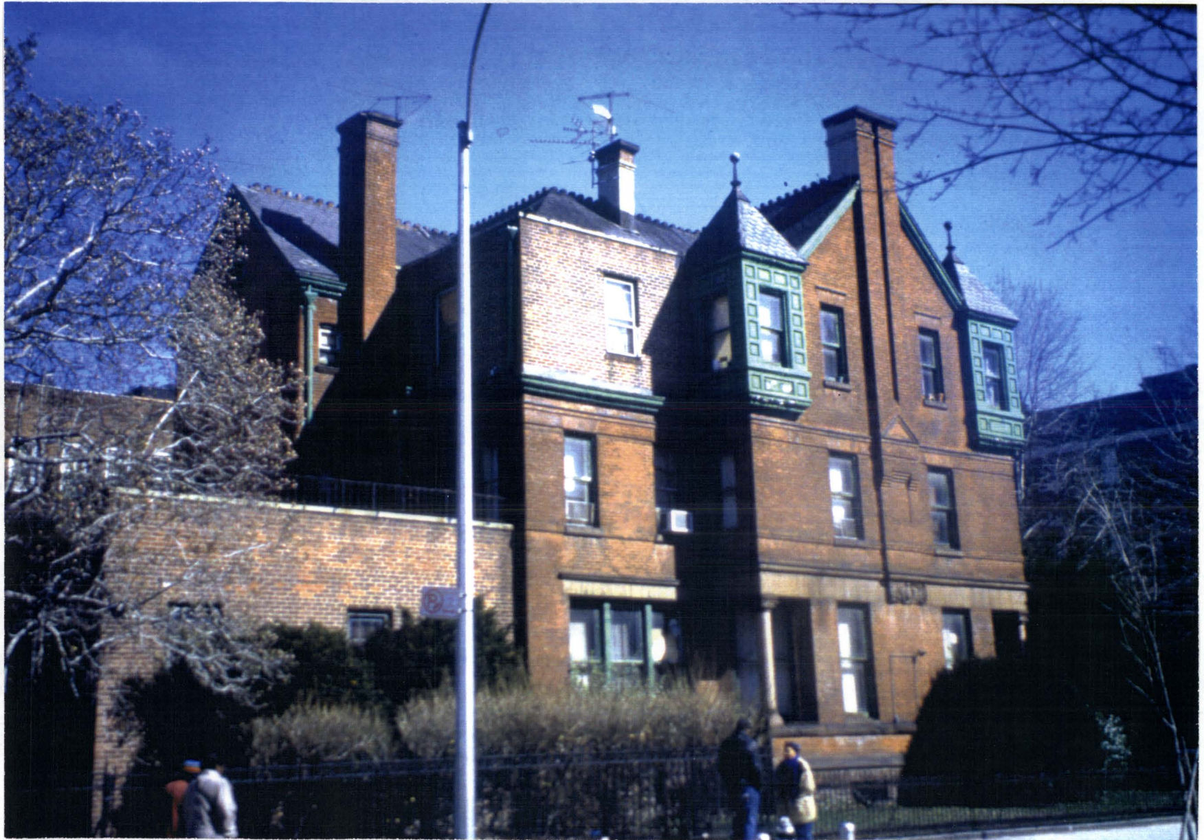
John and Elizabeth Truslow House, 96 Brooklyn Avenue, Brooklyn. View of rear elevation with addition
