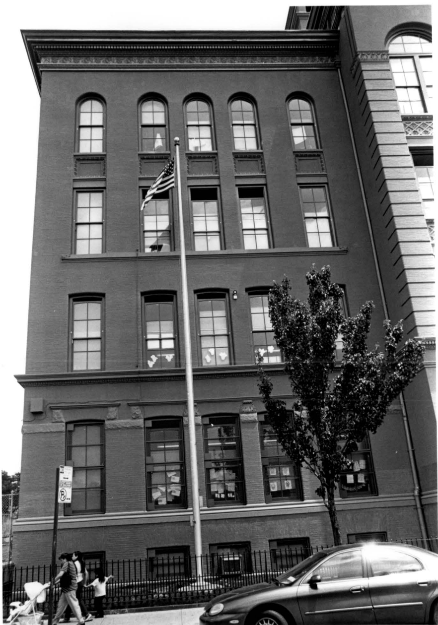
PUBLIC SCHOOL 116 (Elizabeth Farrell School) , 515 Knickerbocker Avenue, Brooklyn. Knickerbocker Avenue facade. Photo: Carl Forster, 2002
