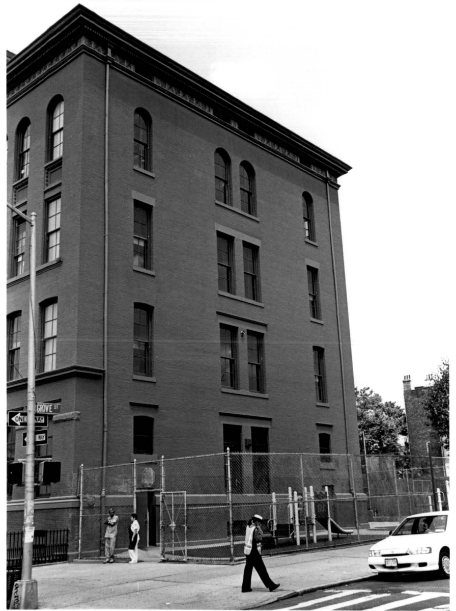
PUBLIC SCHOOL 116 (Elizabeth Farrell School) , 515 Knickerbocker Avenue, Brooklyn. Grove Street facade. Photo: Carl Forster, 2002
