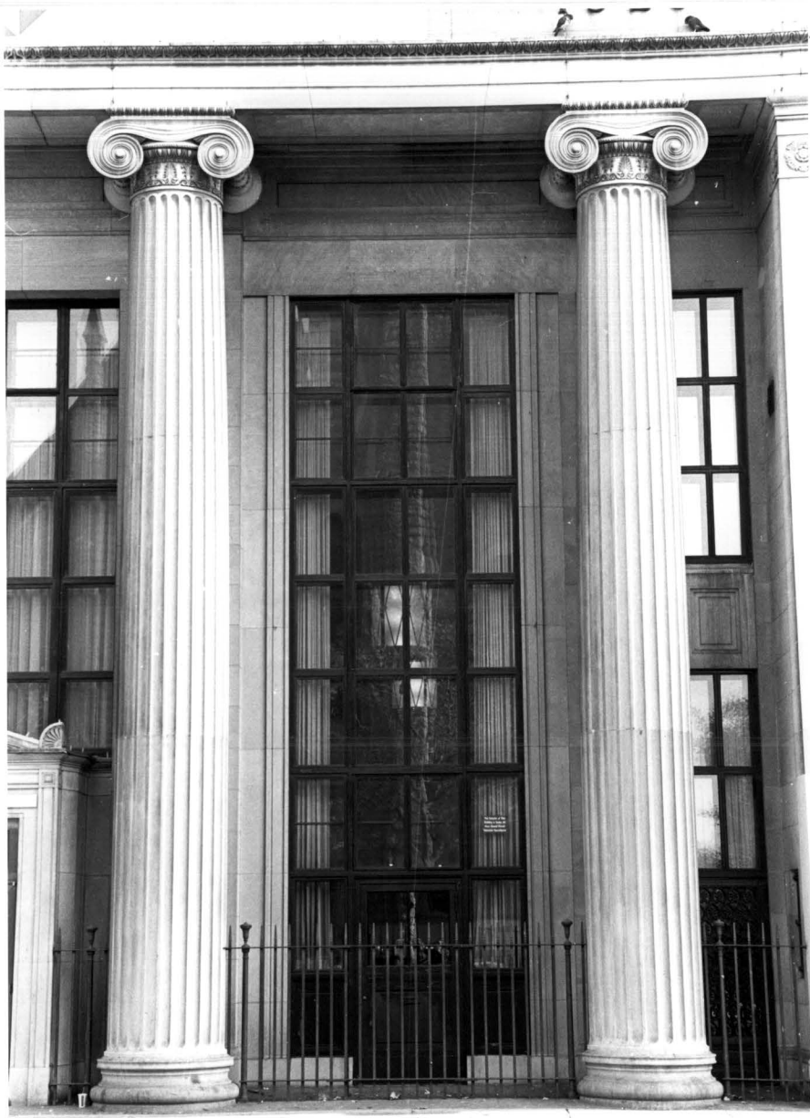
Detail of freestanding Ionic columns facing Amsterdam Avenue. Photo: Carl Foster, 1997
