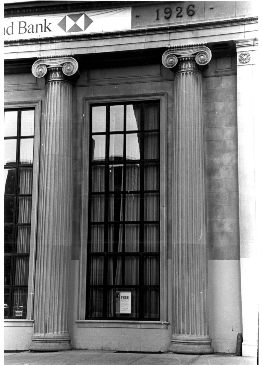
Detail of the engaged columns facing West 96th Street. Photo: Carl Foster: 1997
