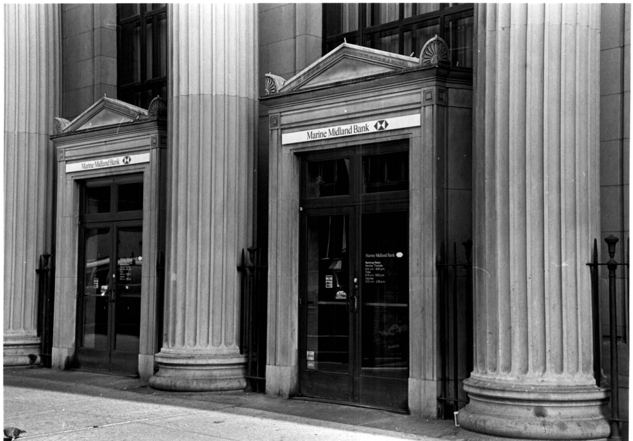
Detail of the paired entrances facing Amsterdam Avenue.
