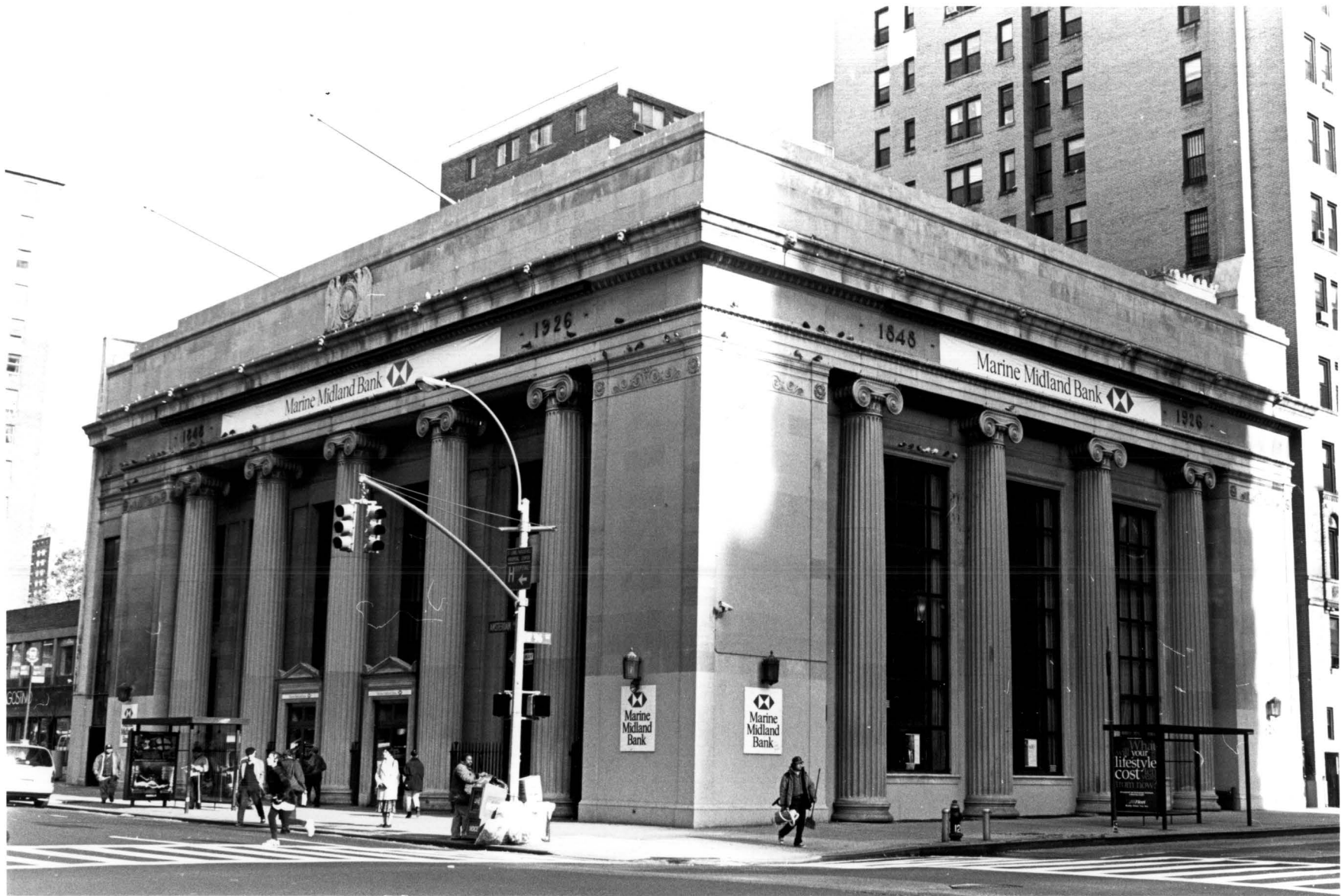
(Former) East River Savings Bank, northeast corner of Amsterdam Avenue and West 96th Street. Photo: Carl Foster, 1997
