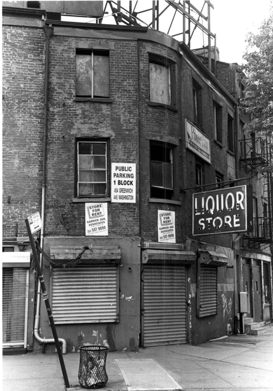
480 Greenwich Street/ 502 Canal Street House, Manhattan Corner section of facade Photo by: Carl Forster, June, 1998
