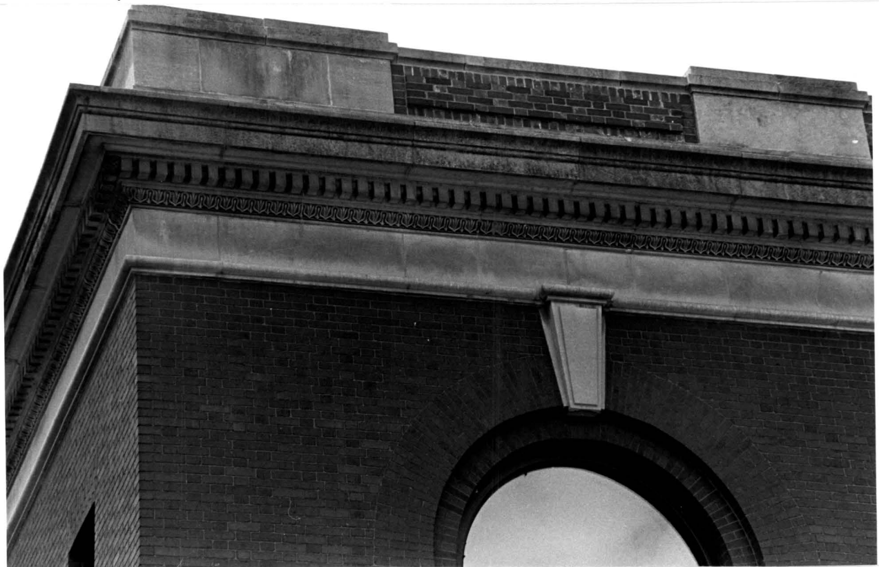
New York Public Library, Morrisania Branch, 610 East 169th Street, The Bronx Detail of cornice and parapet. Photo: Carl Forster, 1998
