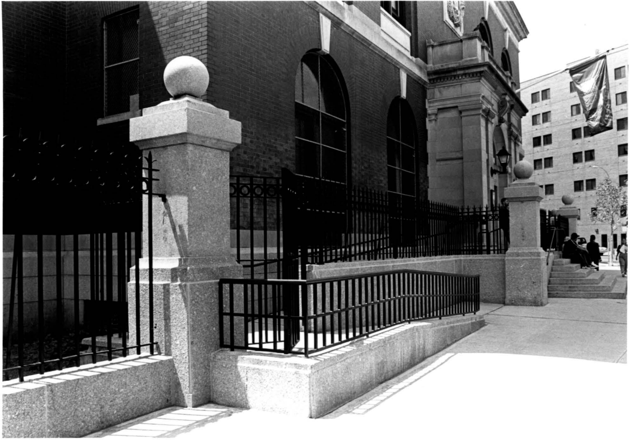
New York Public Library, Morrisania Branch, 610 East 169th Street, The Bronx Handicapped-accessible ramp
