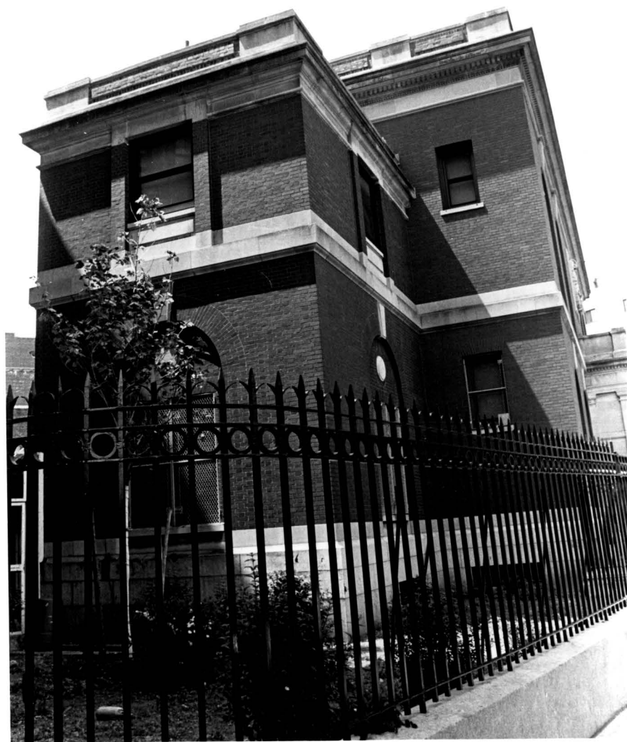
New York Public Library, Morrisania Branch, 610 East 169th Street, The Bronx East wing. Photo: Carl Forster, 1998
