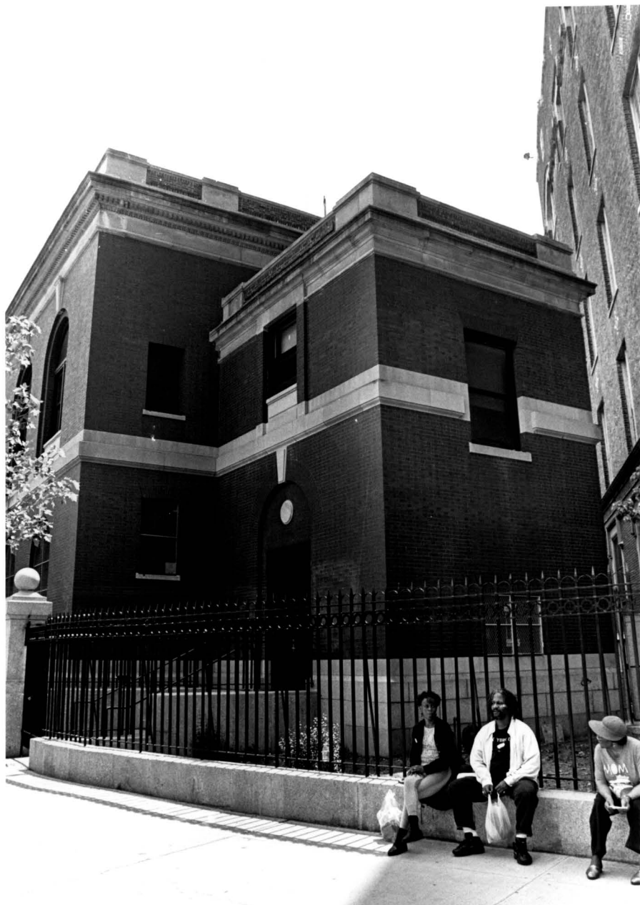
New York Public Library, Morrisania Branch, 610 East 169th Street, The Bronx West wing. Photo: Carl Forster, 1998
