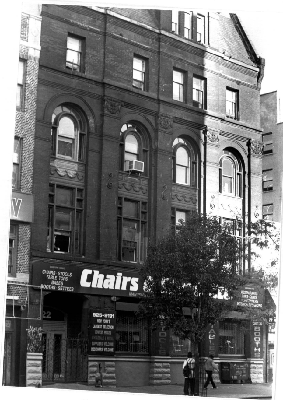
Detail of floors one through four Photo: Joseph Brooks, 1998
