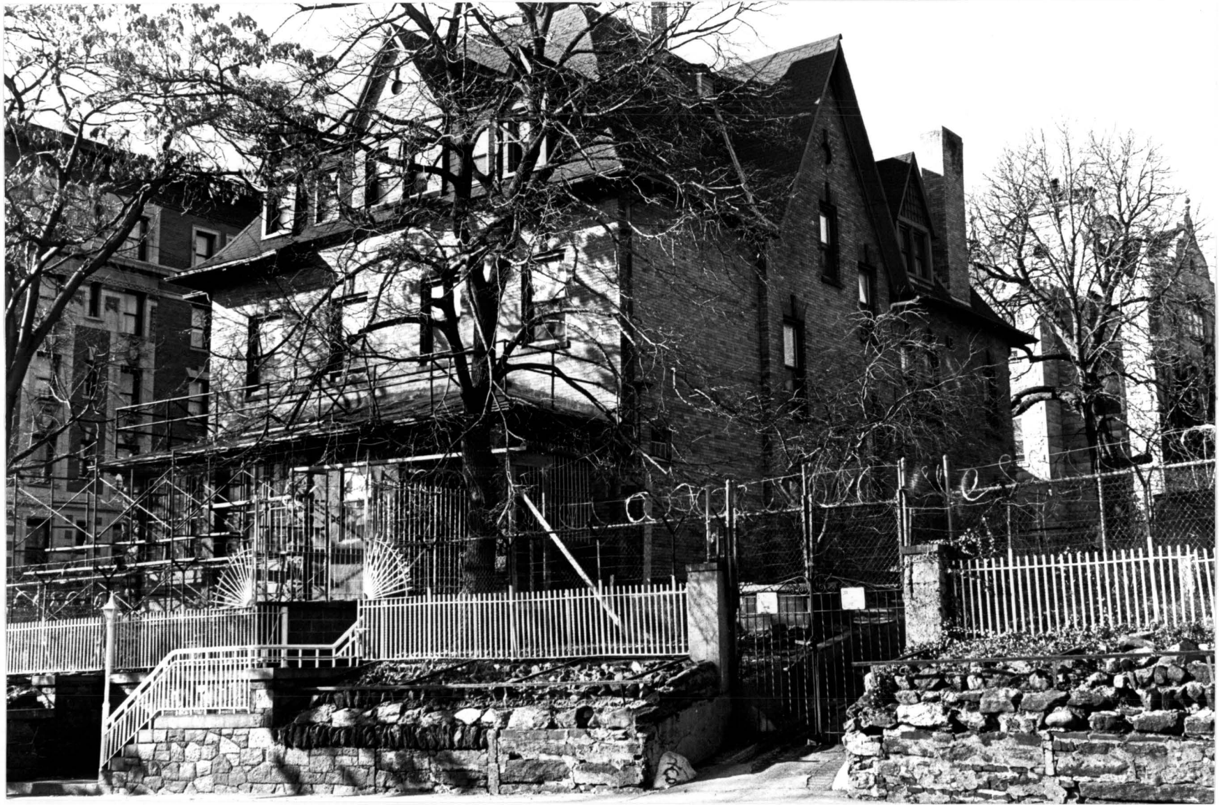
Nicholas C. and Agnes Benziger House, view of north facade Photo: Carl Forster
