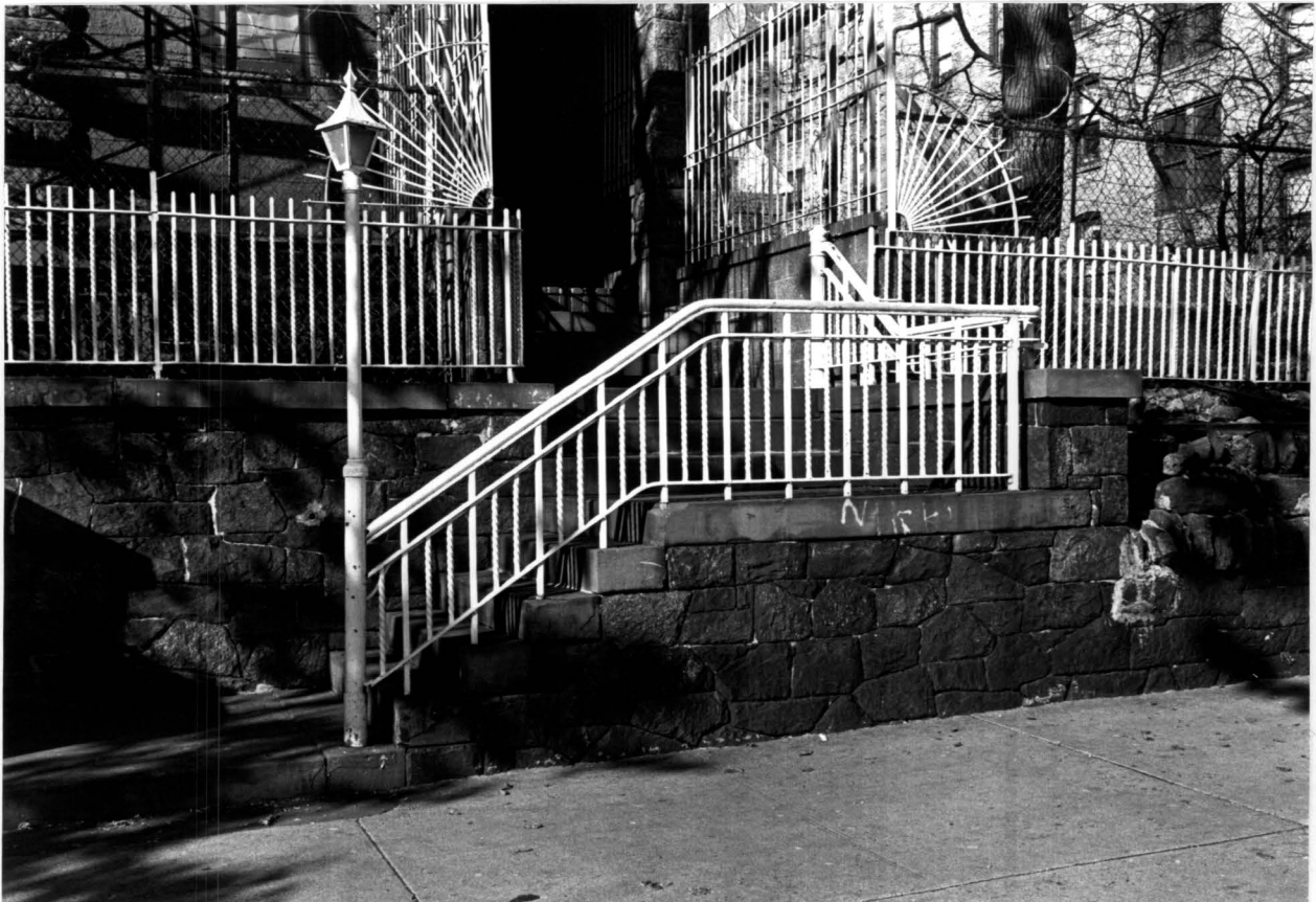
Nicholas C. and Agnes Benziger House Edgecombe Avenue stairs, railing, and fence
