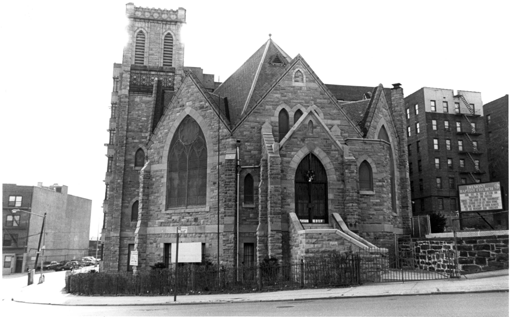
Tremont Baptist Church, 324 East Tremont Avenue, Borough of the Bronx.
