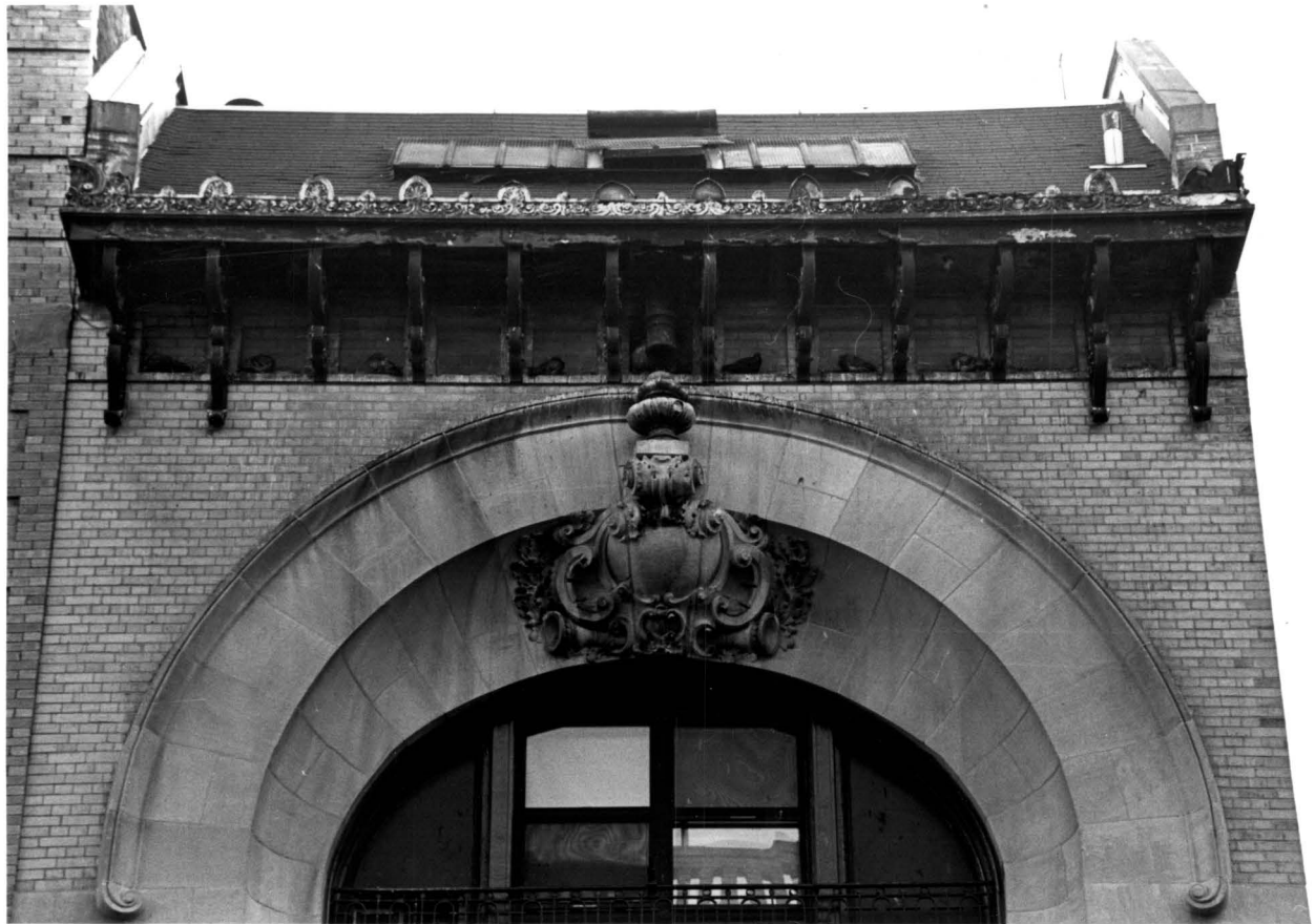
Fire Engine Company 67 514 West 170 th Street, Manhattan Cornice Details Photo: Carl Forster
