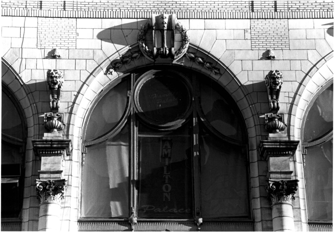
(Former) Hamilton Theater, 3560-3568 Broadway, Manhattan. Detail at third story.
