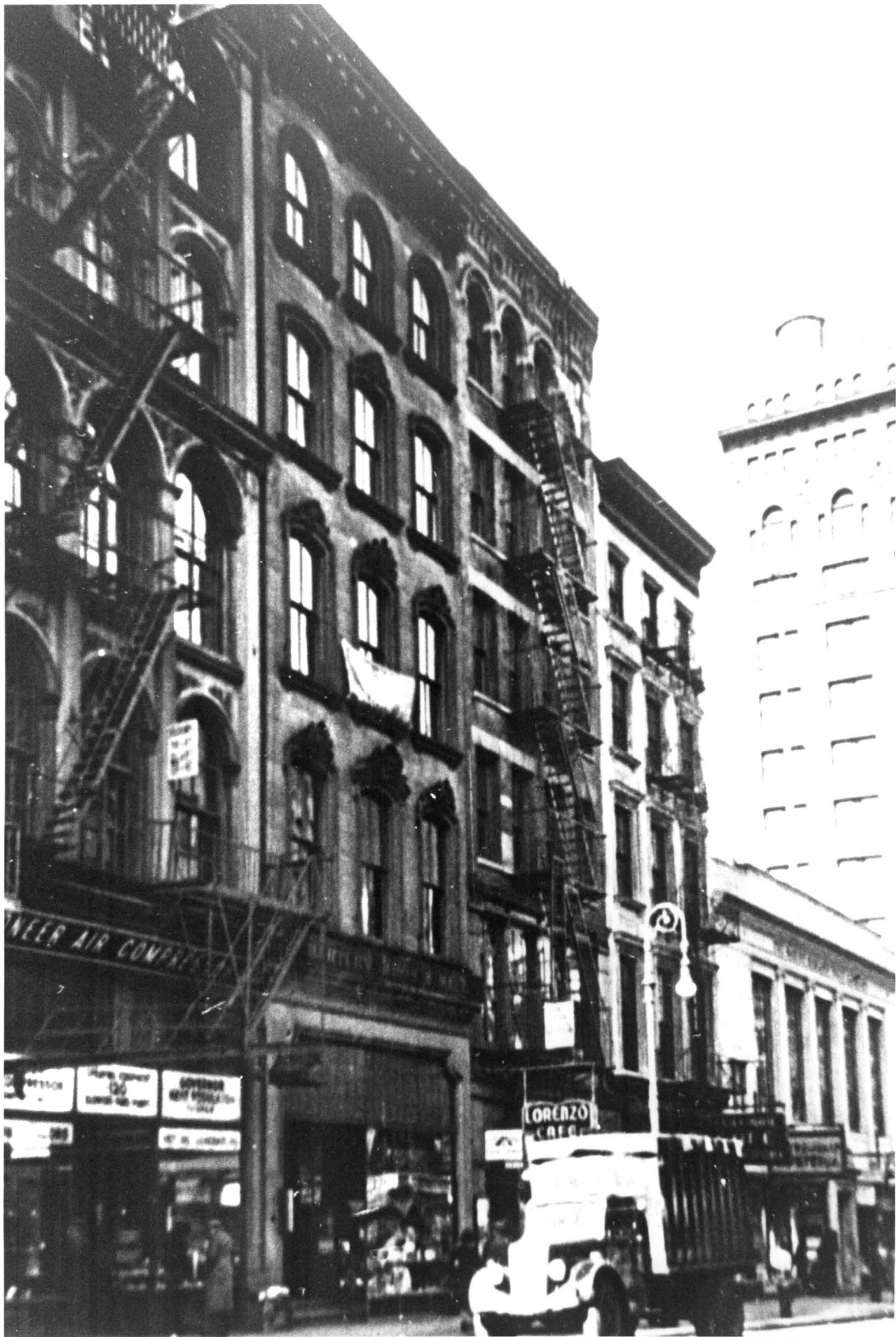
Swift, Seaman & Co. Building, 122 Chambers Street elevation Photo: New York City Dept. of Taxes (c. 1938), Municipal Archives
