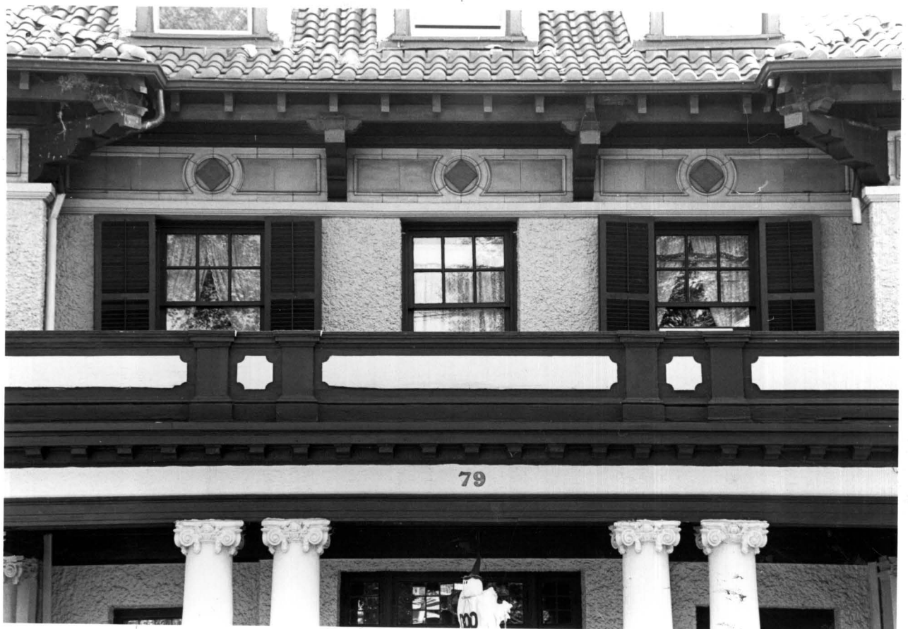
Louis A. and Laura Stirn House Details of the western entrance facade facing Howard Avenue Photos: Carl Forster
