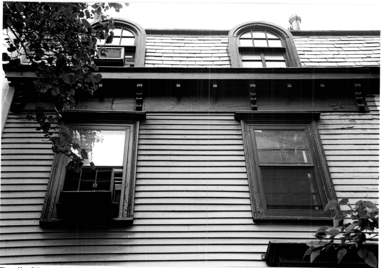
Detail of Second Floor Windows and Mansard Roof
