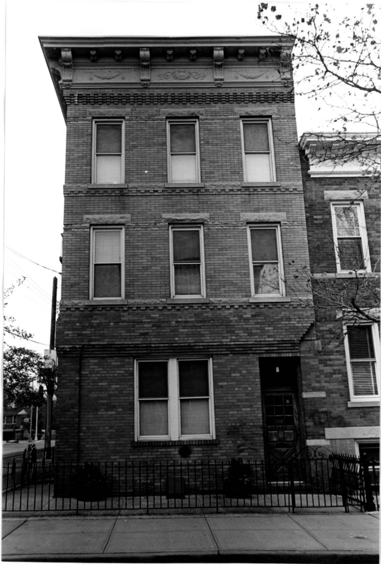
1896 Stockholm Street (Stockholm Street Facade) Photo: Carl Forster, 2000
