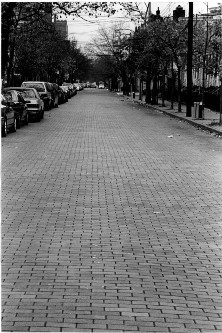
Brick Pavement, looking South Photo: Carl Forster, 2000
