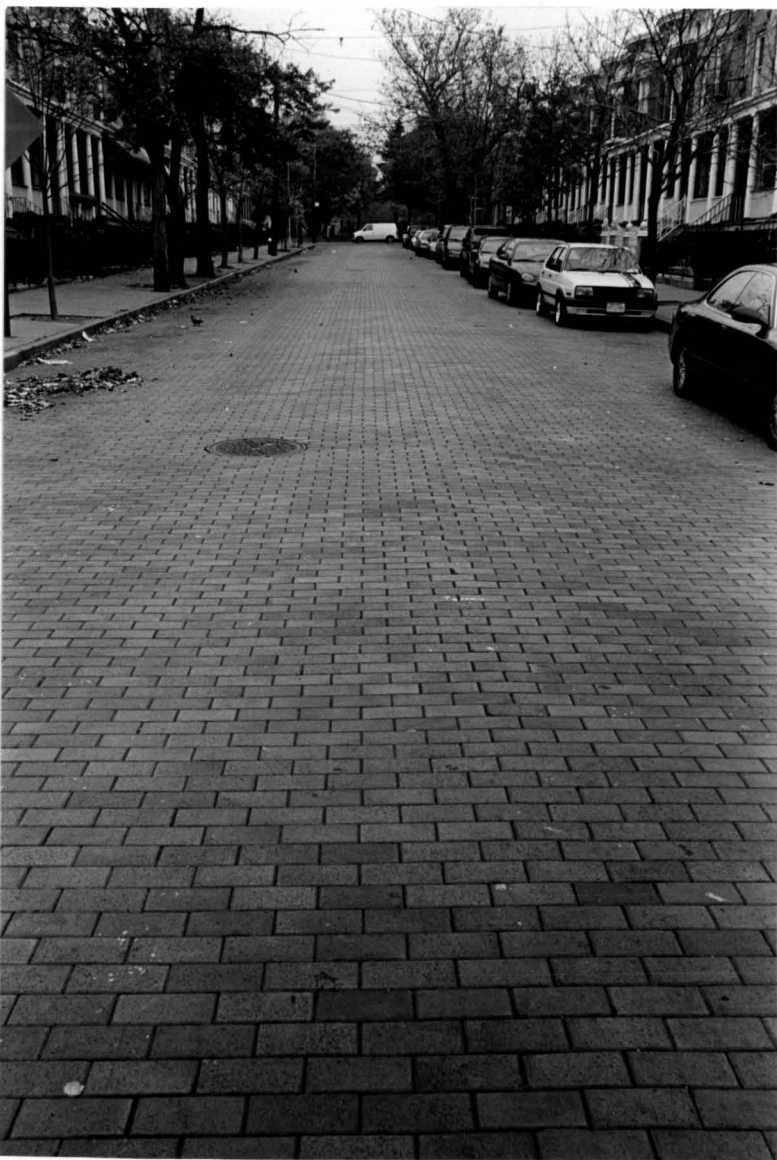
Brick Pavement, looking North Photo: Carl Forster, 2000
