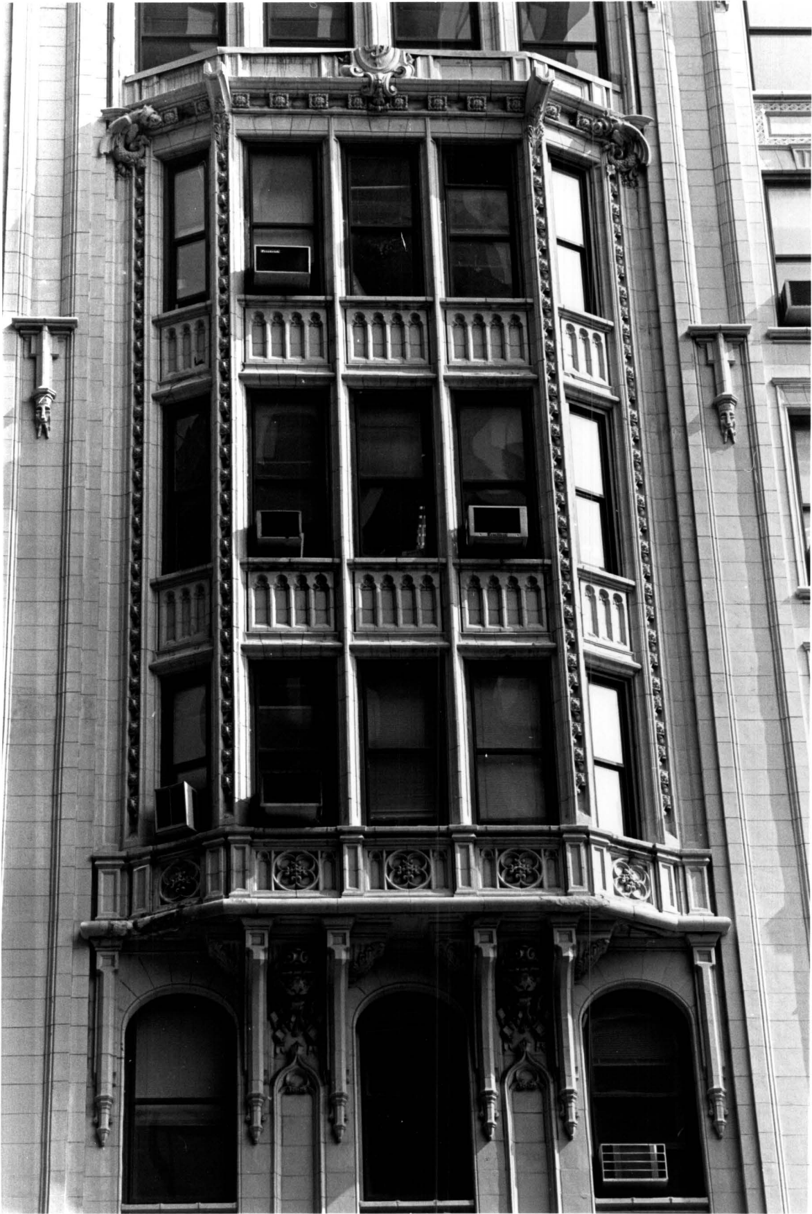
A.T. Demarest & Co. and Peerless Motor Car Co. Buildings (later General Motors Corp. Building) Broadway facade oriel detail
