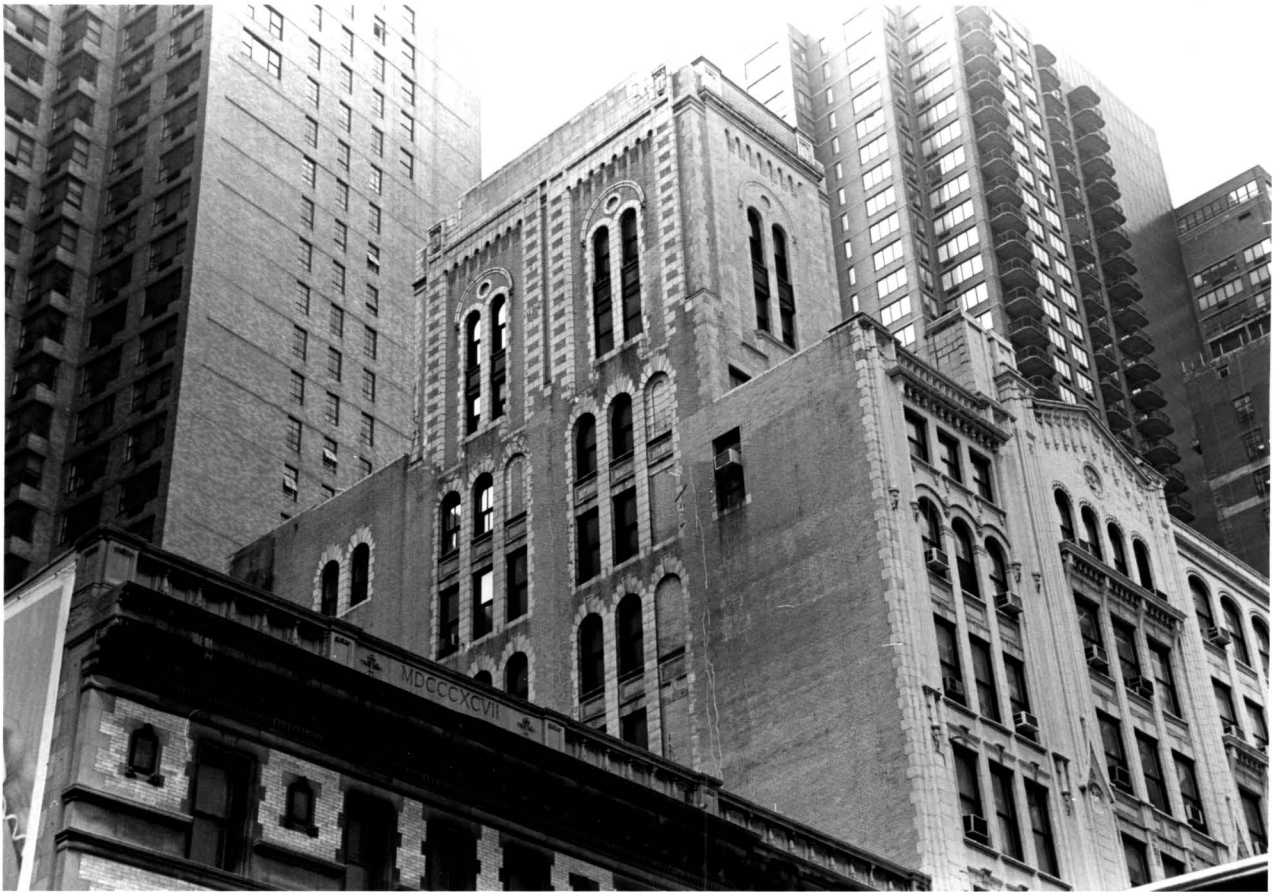
A.T. Demarest & Co. and Peerless Motor Car Co. Buildings (later General Motors Corp. Building) Tower details
