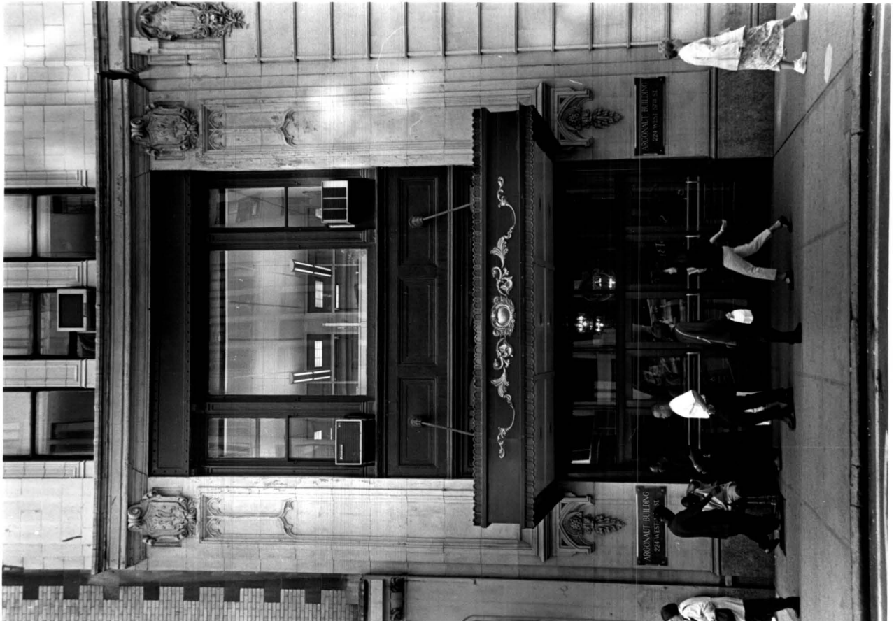
A.T. Demarest & Co. and Peerless Motor Car Co. Buildings (later General Motors Corp. Building) West 57 th Street entrance (left) and Corner entrance (right) Photos: Carl Forster
