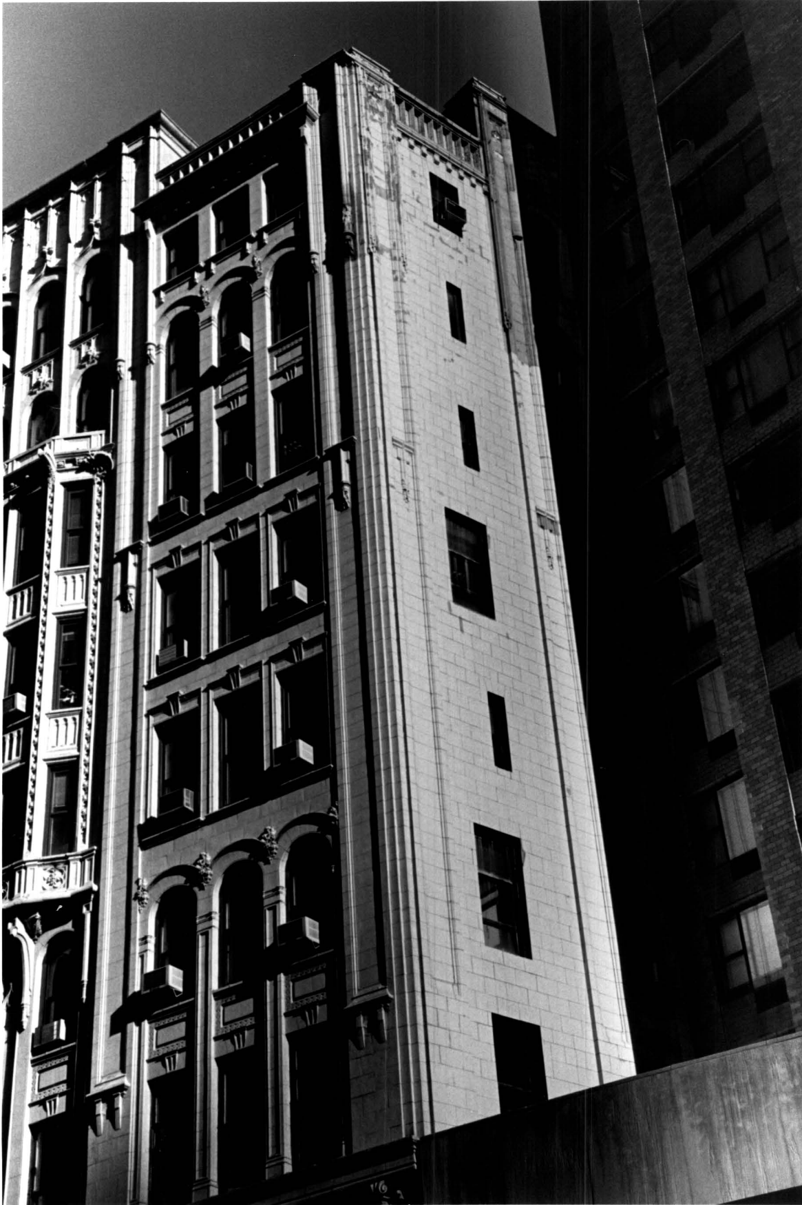
A.T. Demarest & Co. and Peerless Motor Car Co. Buildings (later General Motors Corp. Building) South facade
