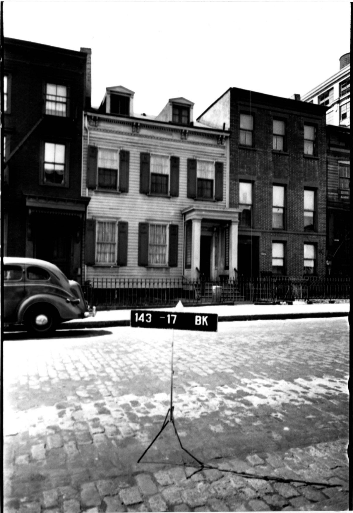
186 Duffield Street House at its former location at 108 Johnson Street "Tax" Department Photograph, c. 1940 Photo source: NYC Municipal Archives
