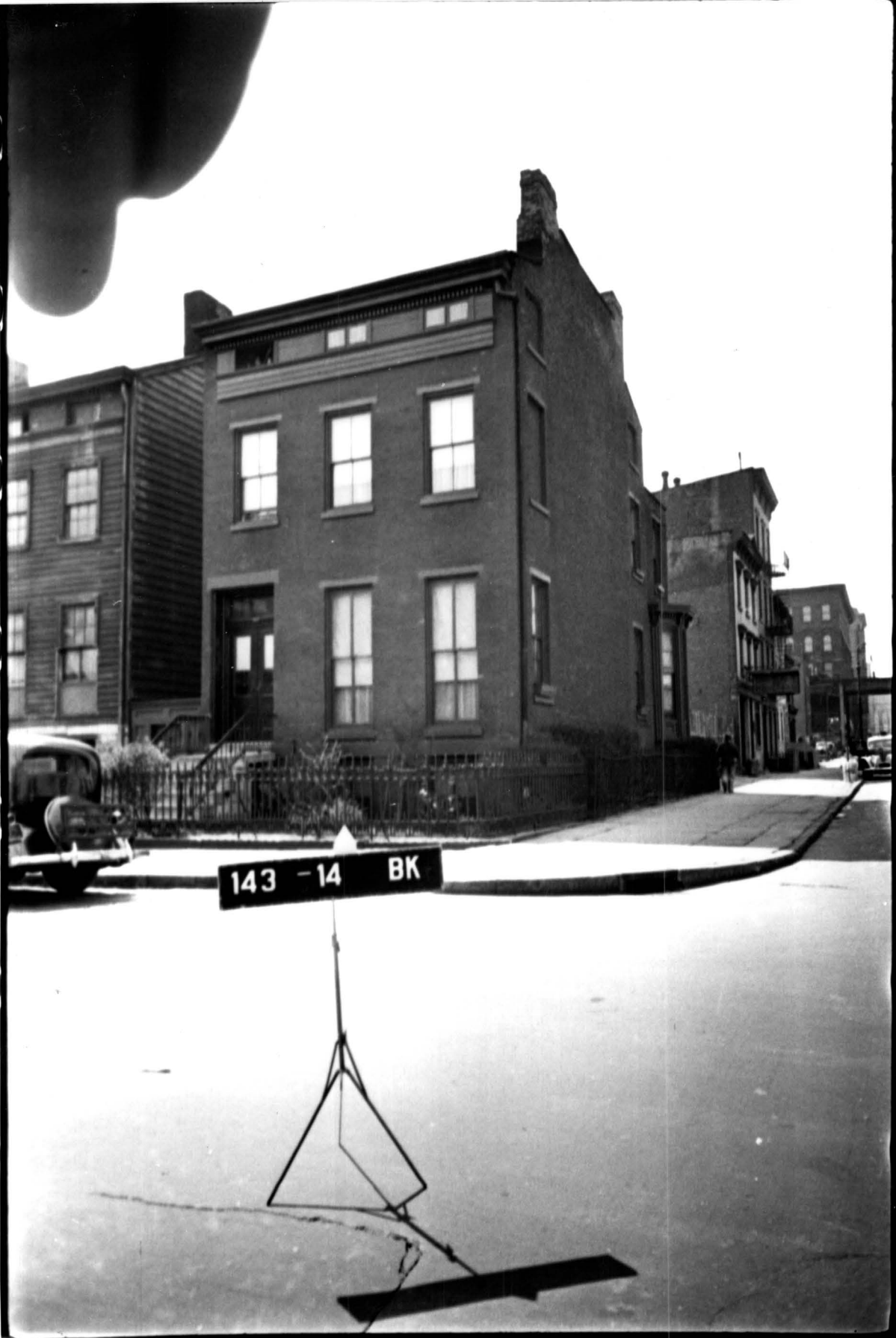
182 Duffield Street House at its former location at 100 Johnson Street "Tax" Department Photograph, c. 1940 Photo source: NYC Municipal Archives
