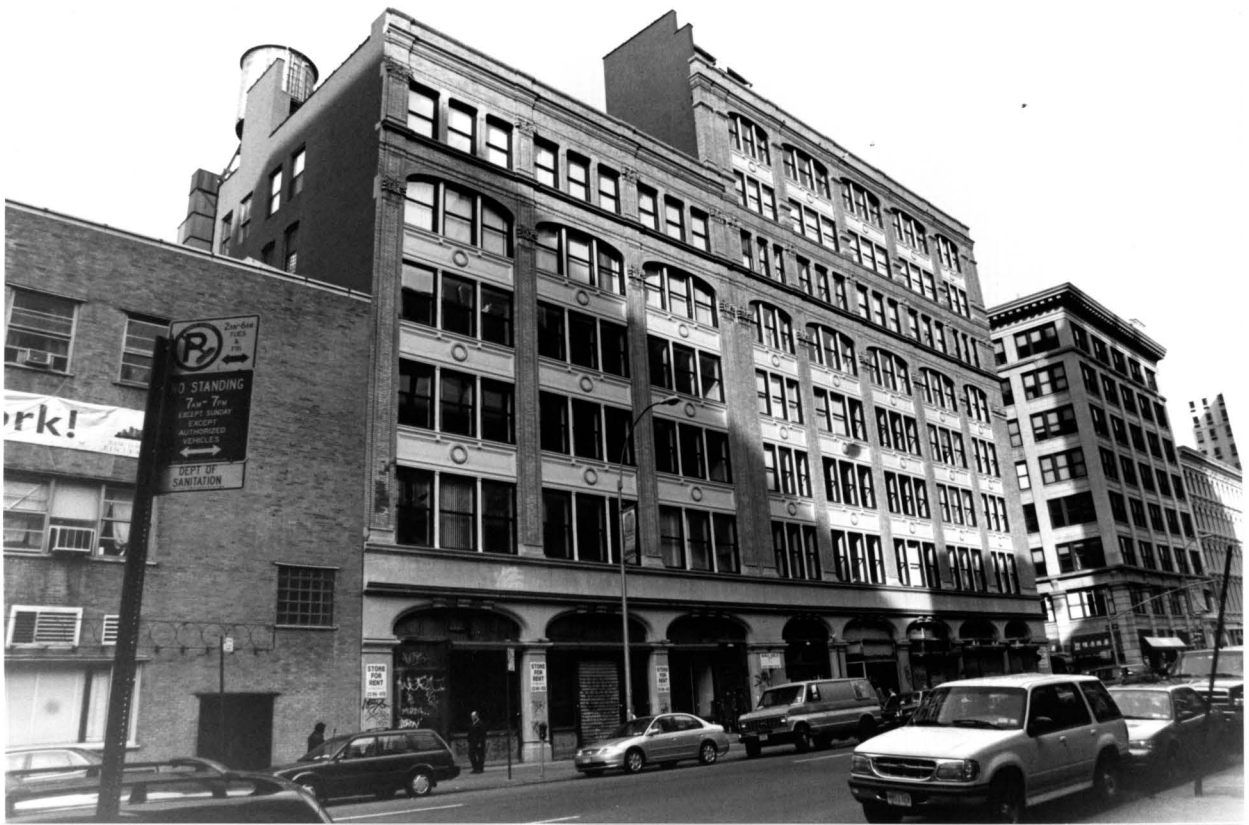
Lafayette Street Facade
