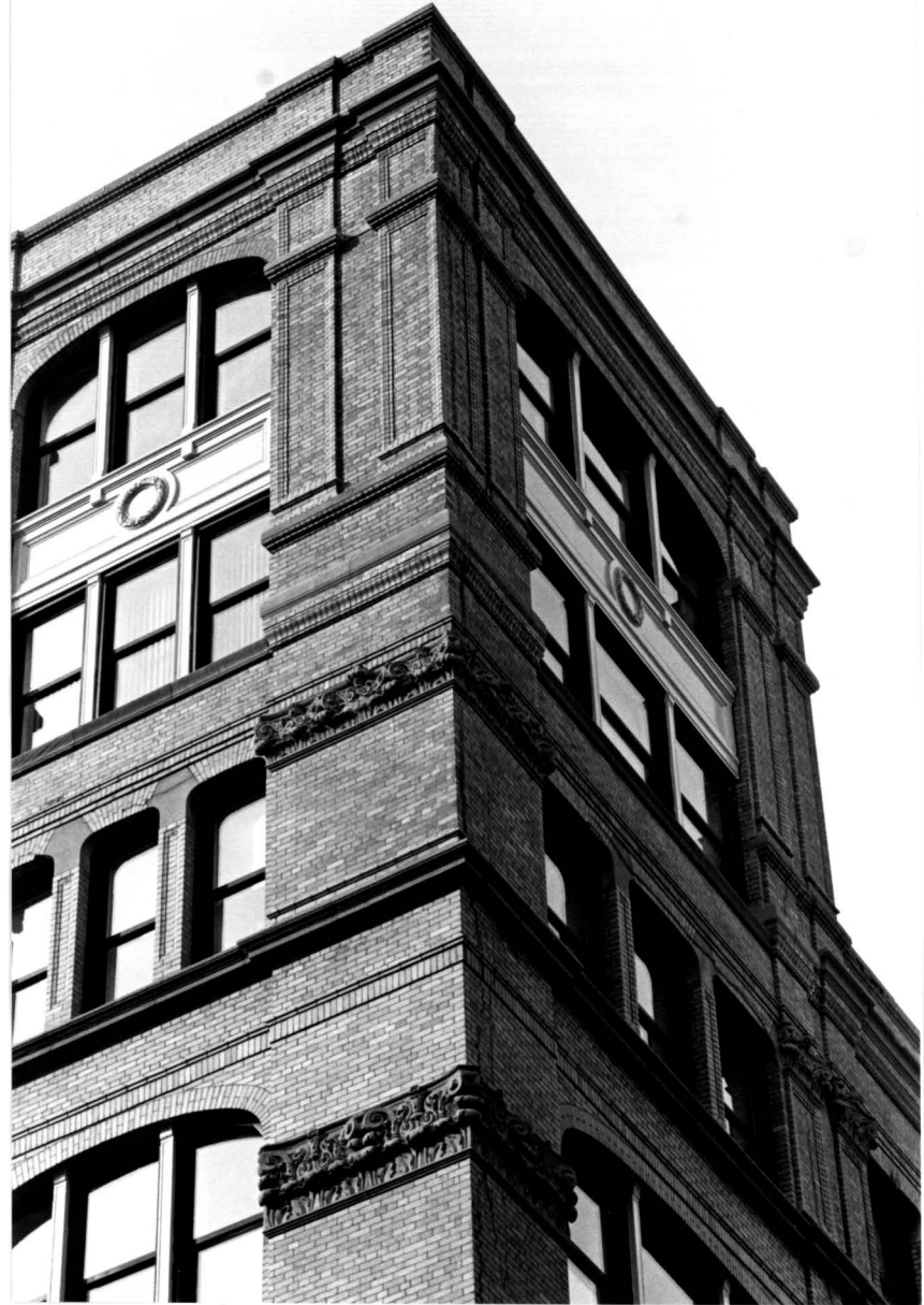
94-100 Lafayette Street Building Detail of Corner Photo: Carl Forster
