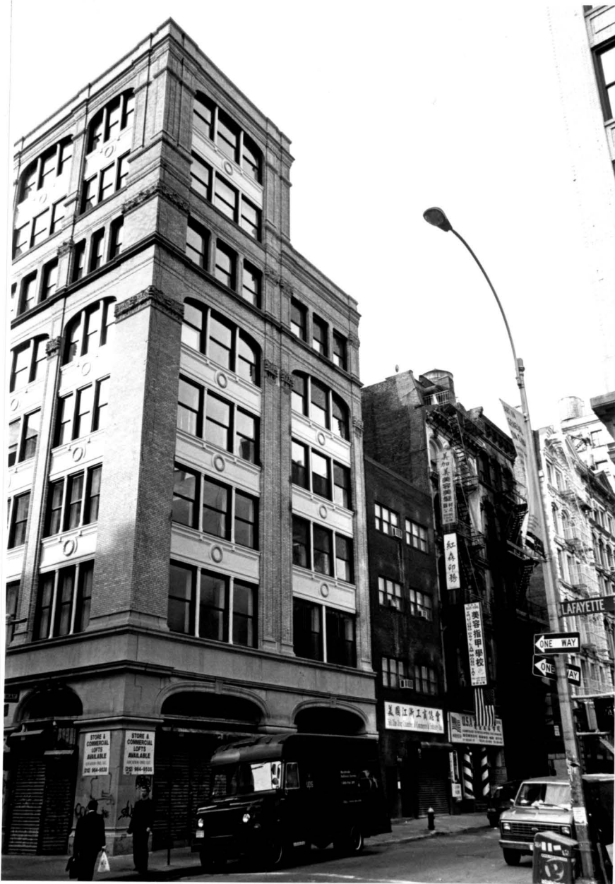
94-100 Lafayette Street Building Walker Street Facade Photo: Carl Forster
