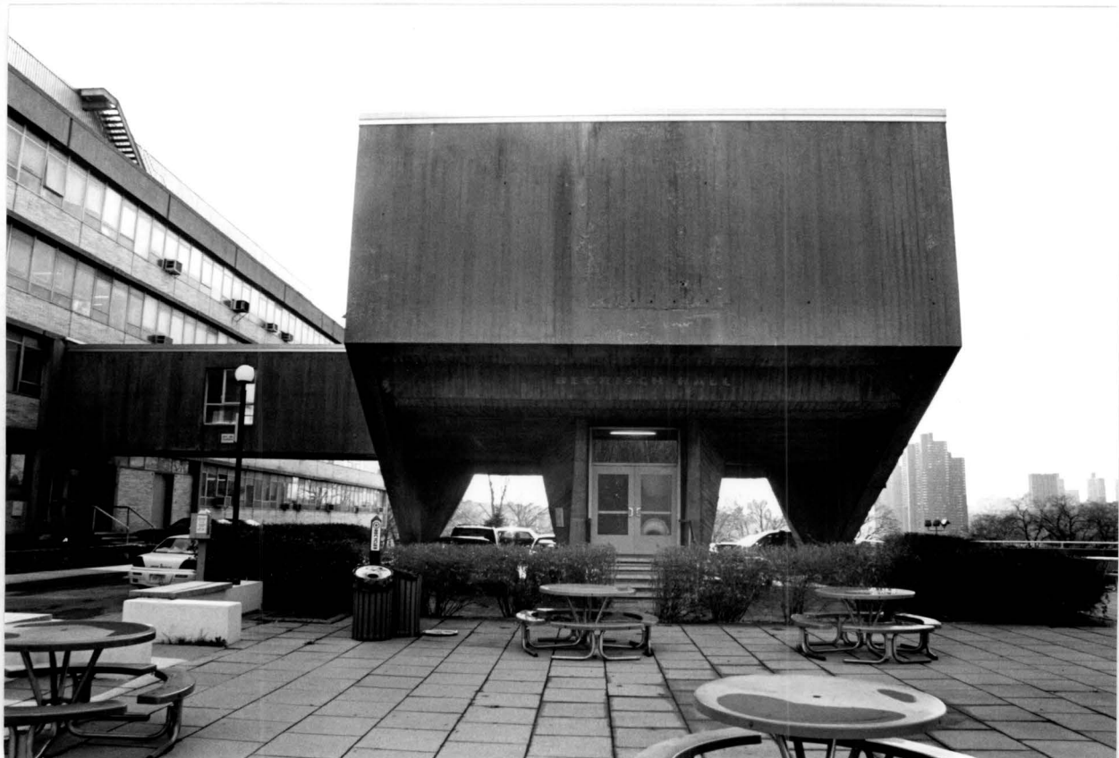
Begrish Hall, north facade, enclosed bridge to east Photo: Carl Forster
