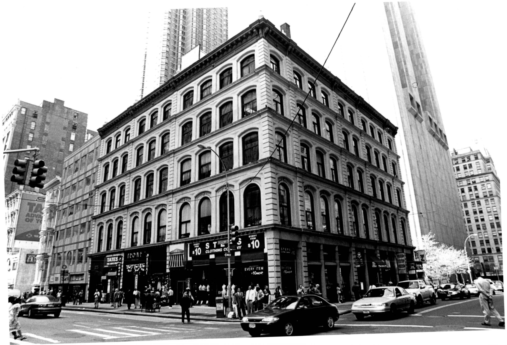
325-333 Broadway Building, 325-333 Broadway (aka 90 Worth Street), Manhattan View from the northeast showing the Broadway and Worth Street facades Photo: Carl Forster
