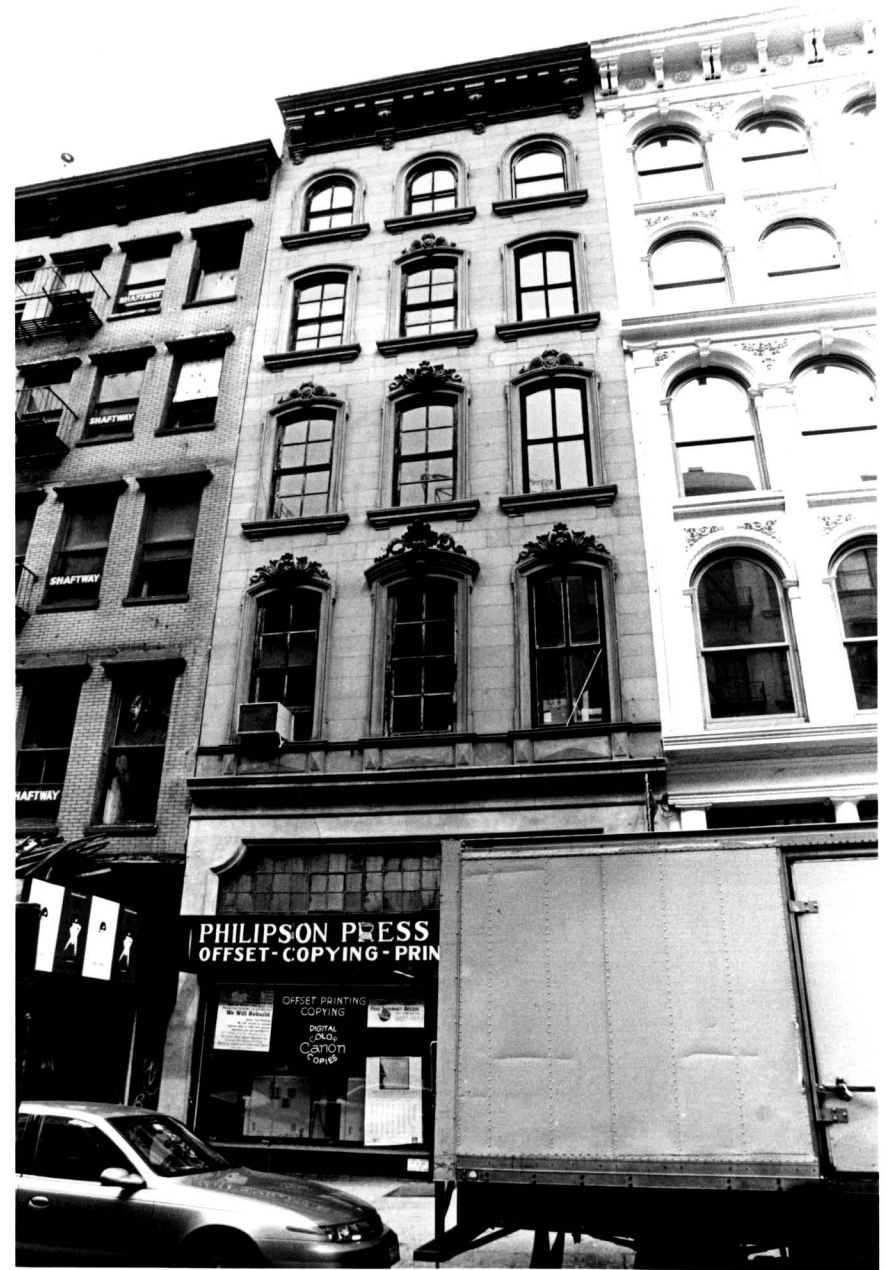
No. 52 Warren Street, aka 120 Chambers Street, built c. 1857-58.
