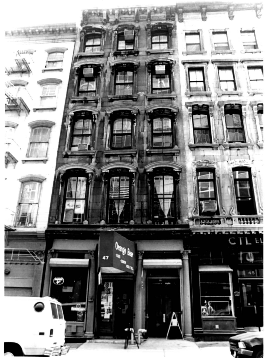
No. 47 Murray Street, built c.1855, attributed to architect Joseph C. Wells.
