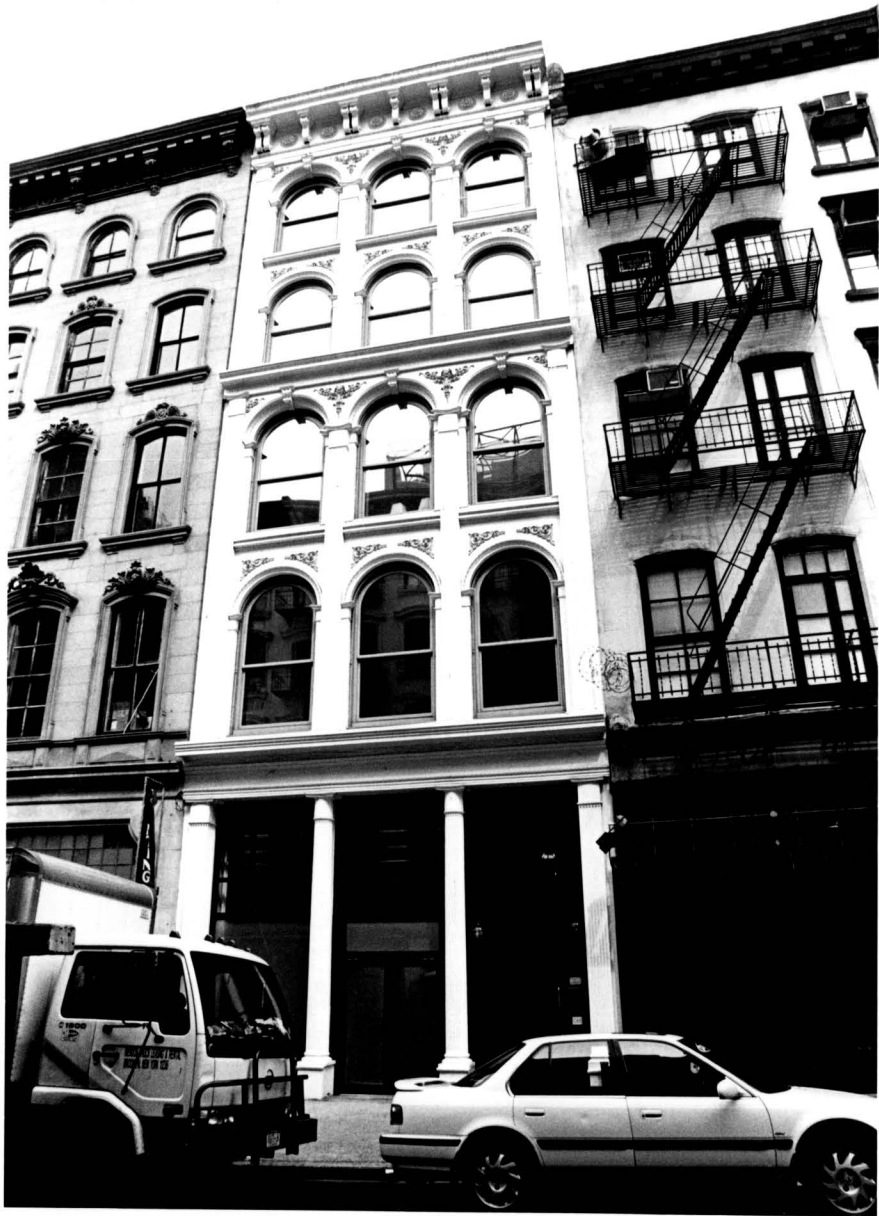
No. 50 Warren Street, built c. 1857-58.
