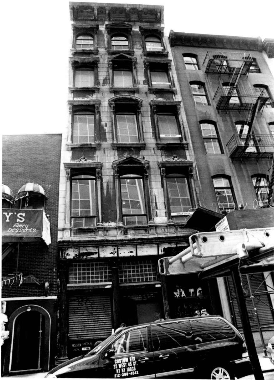
No. 55 Murray Street, built c.1854.
