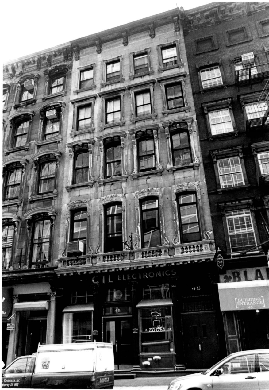
No. 45 Murray Street, built c.1854-55.
