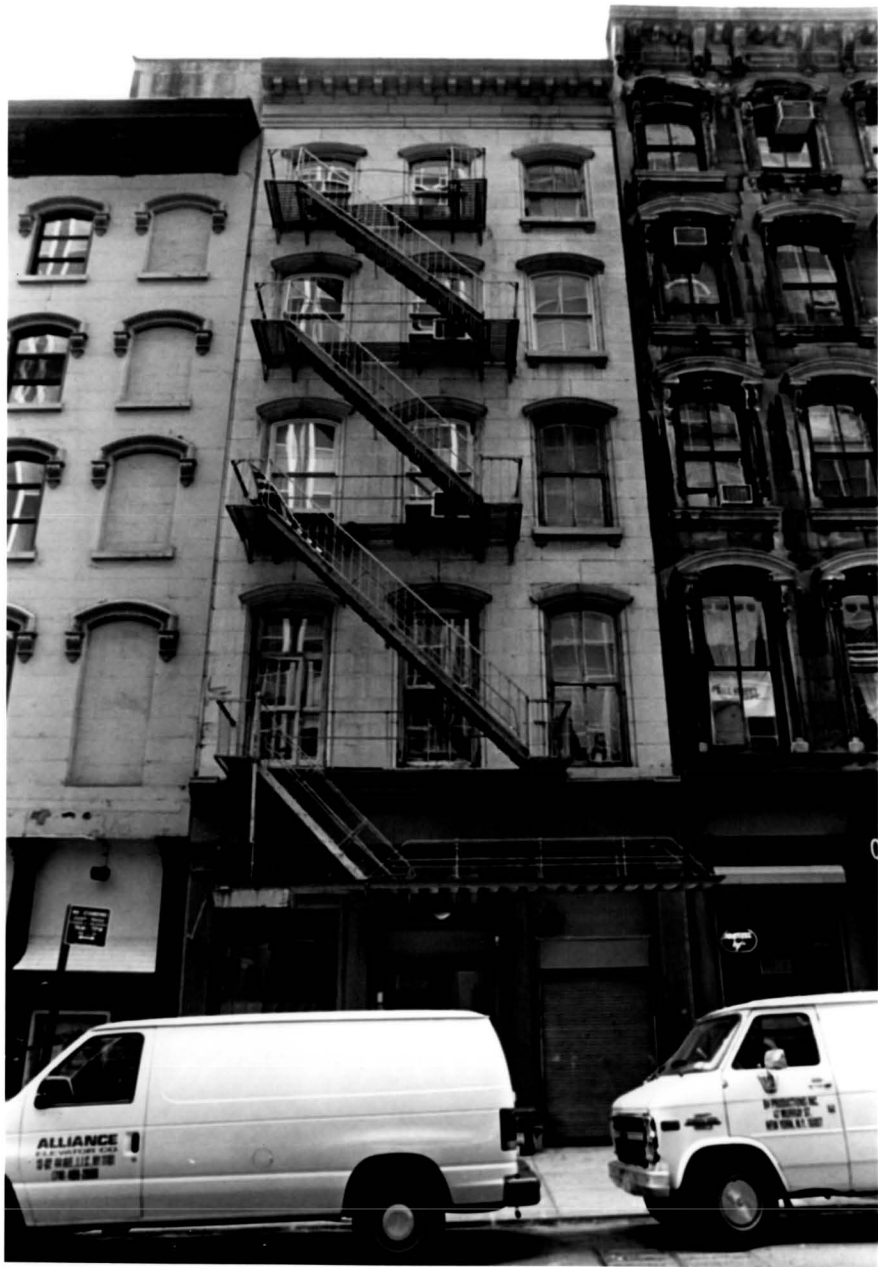
No. 49 Murray Street, built c.1858.
