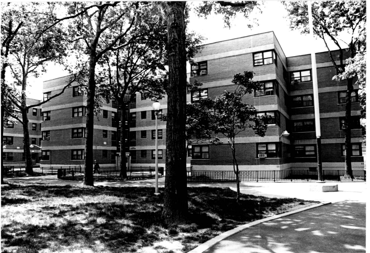
Williamsburg Houses East facade of Building No. 11 Photos by Carl Forster
