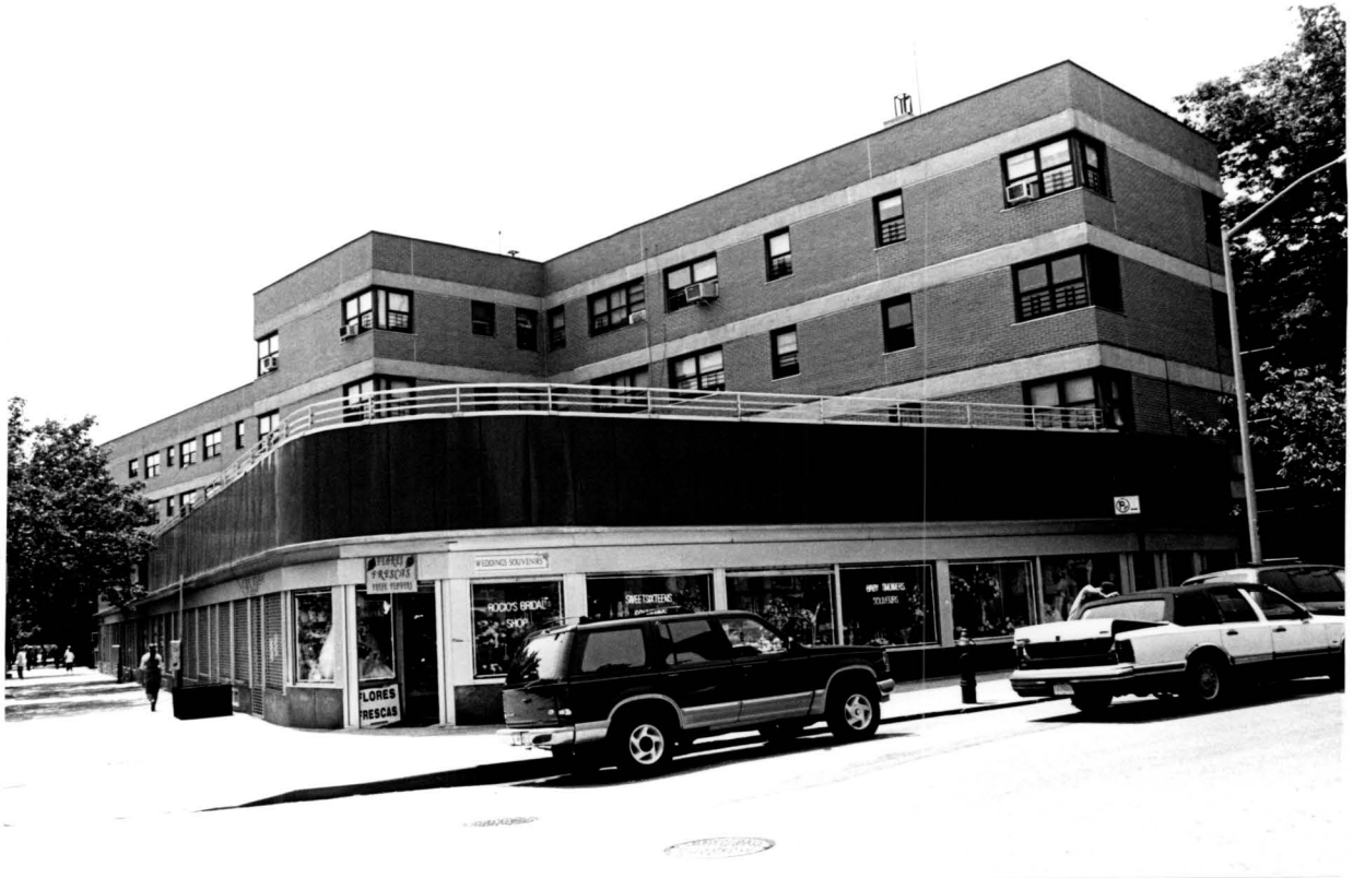
Williamsburg Houses Storefront at Maujer Street and Graham Avenue, part of Building No. 8
