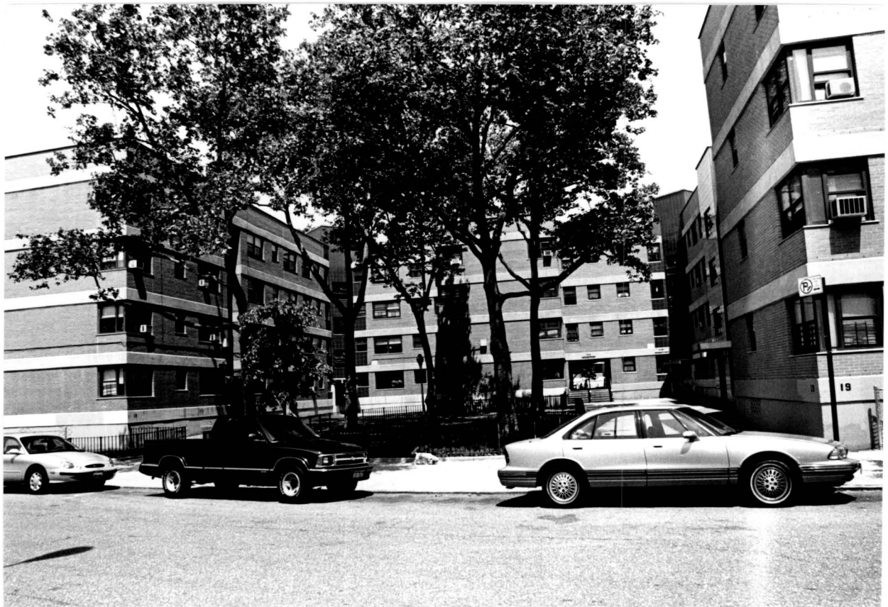
Williamsburg Houses Scholes Street, near Humbolt Street (Building No. 19) Photos by Carl Forster
