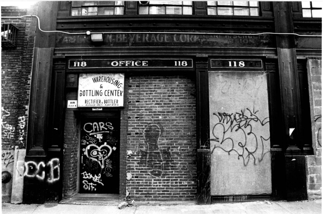
Hecla Iron Works Building first story, east end Photo: Carl Forster
