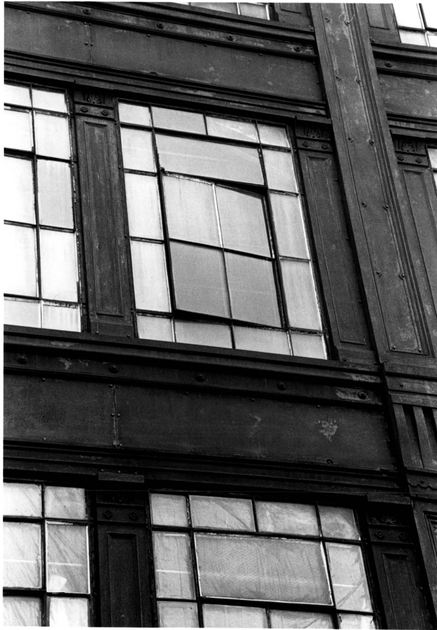
Hecla Iron Works Building windows and pilasters Photo: Carl Forster
