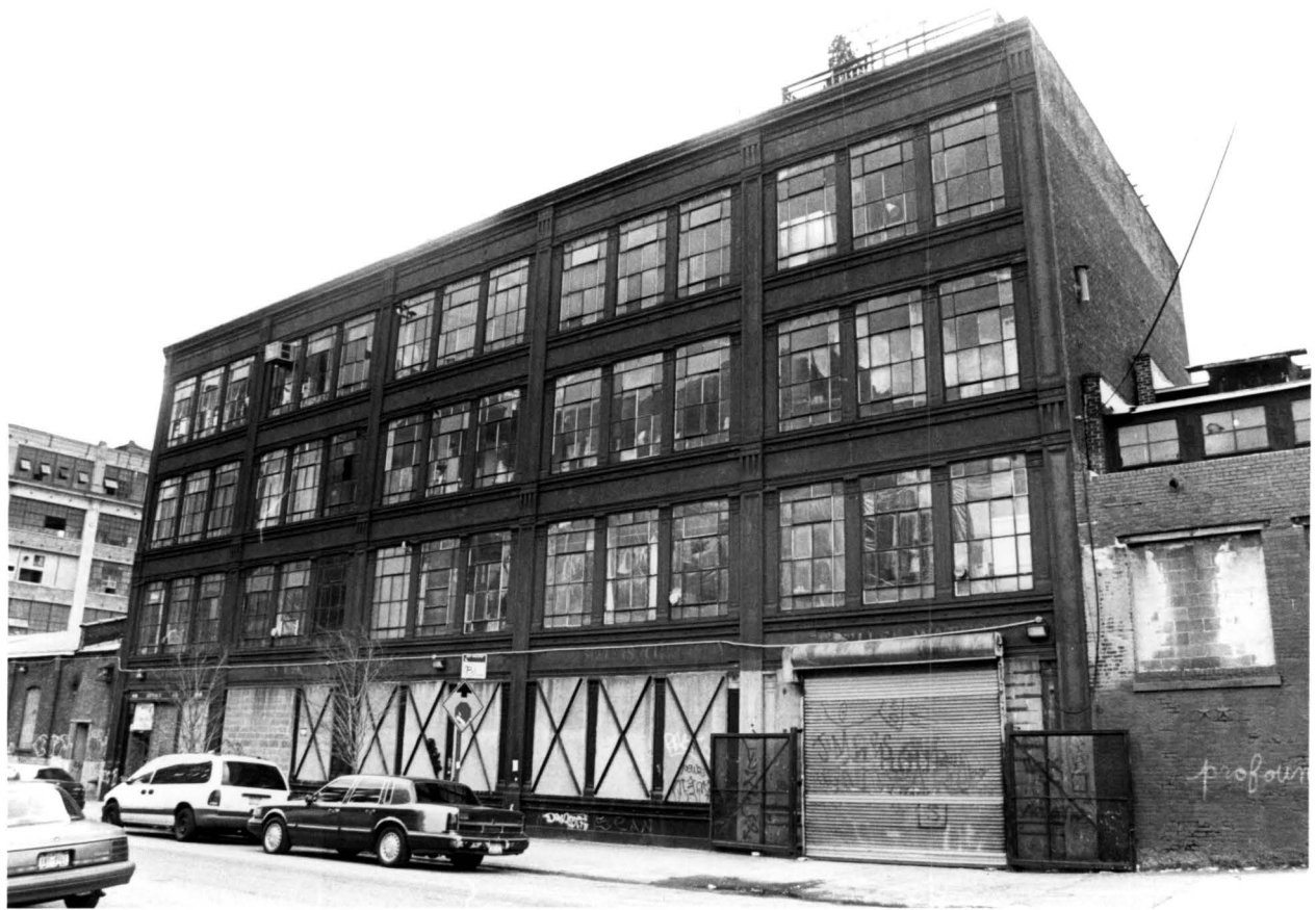
Hecla Iron Works Building 100-118 North 11 th Street, Brooklyn Photo: Carl Forster
