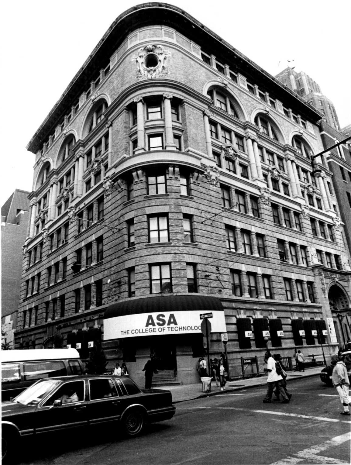
(Former) New York and New Jersey Telephone and Telegraph Building 81 Willoughby Street (aka 119-127 Lawrence Street), Brooklyn
