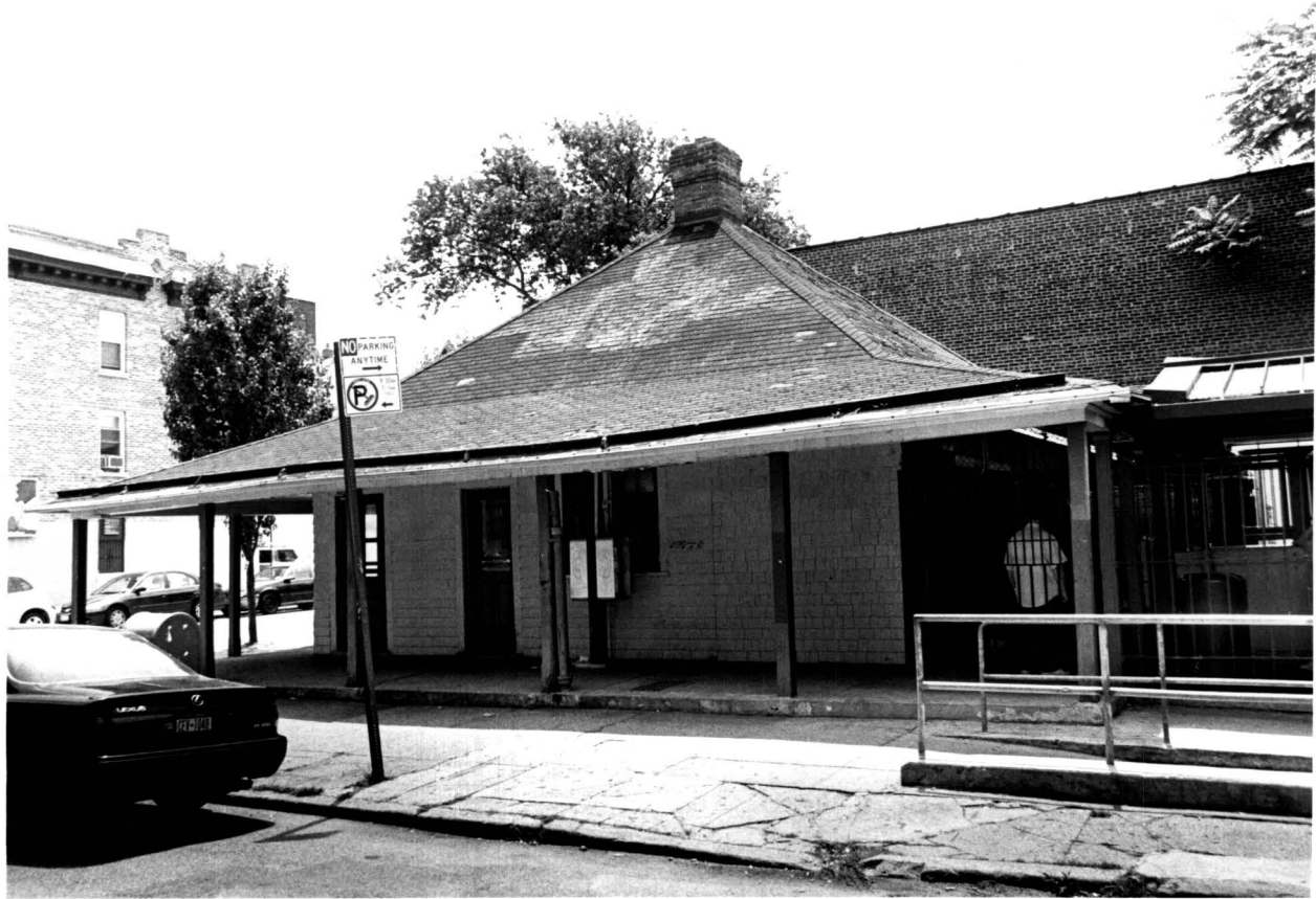
Avenue H Station House Avenue H Facade Photo: Carl Foster, 2004
