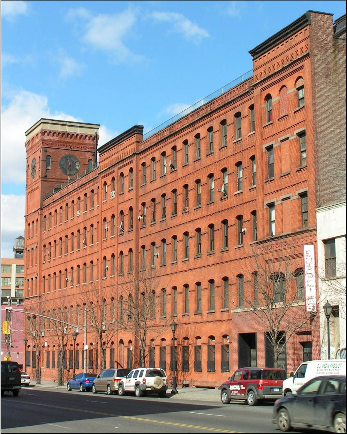
Estey Piano Company Factory, Bruckner Boulevard façade. Photo: Michael Caratzas
