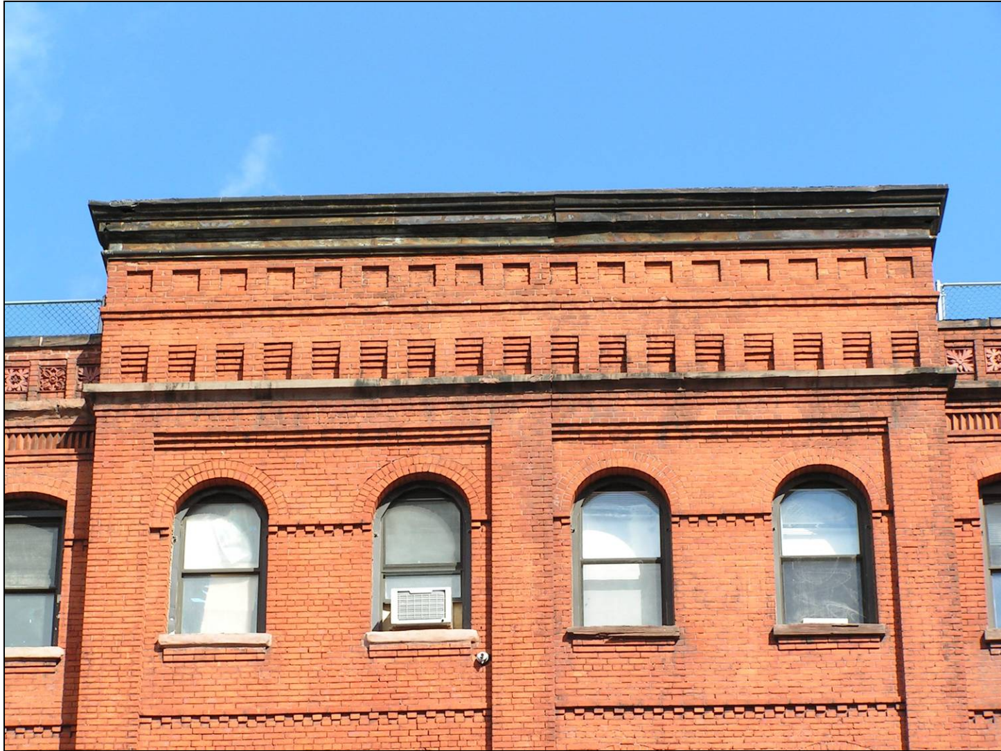
Estey Piano Company Factory, parapet. Photo: Michael Caratzas
