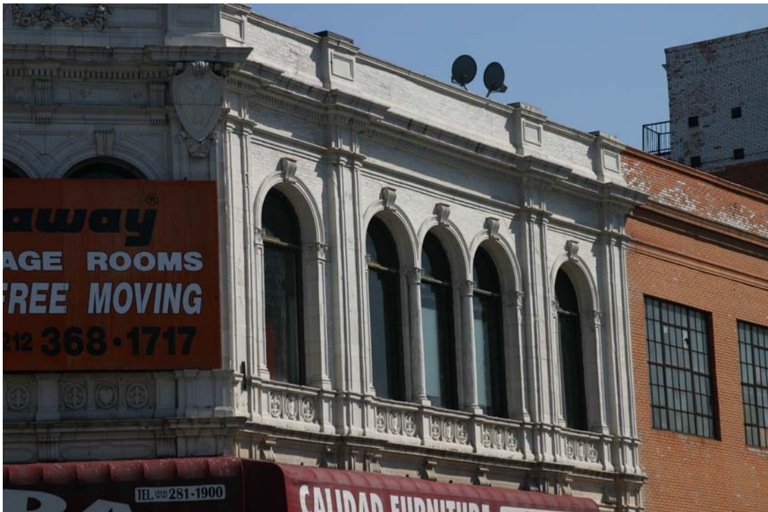
Claremont Theater Building Broadway façade, second story Photos by Carl Forster
