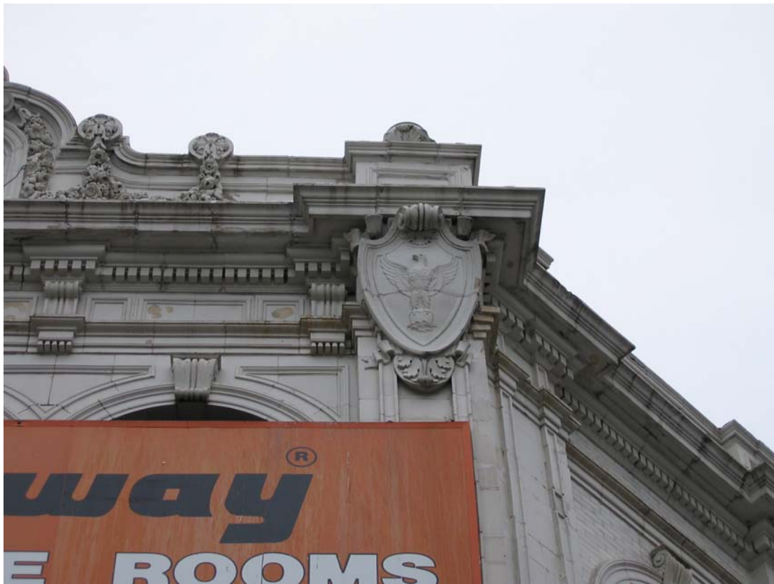
Claremont Theater Building Details: Northwest corner, second story Photos by Carl Forster
